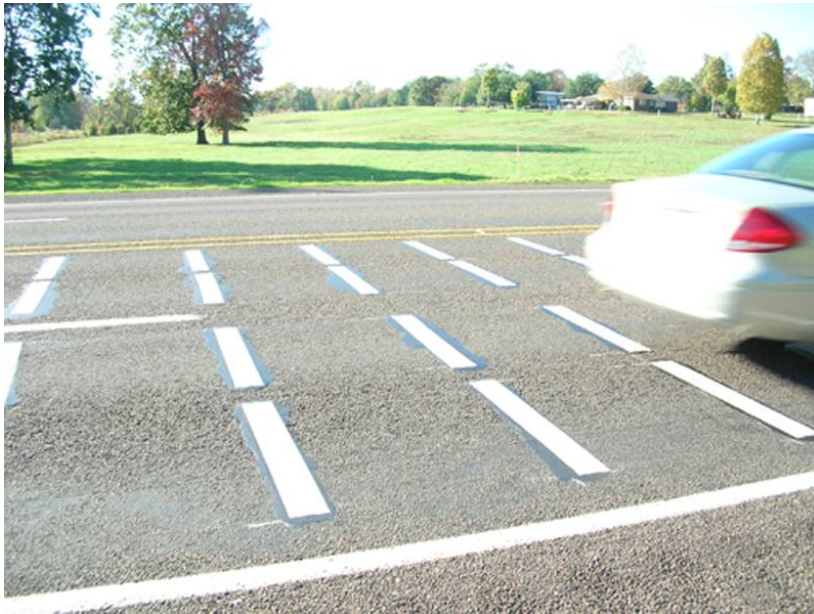
Figure 21 Thermoplastic Transverse Rumble Strips
