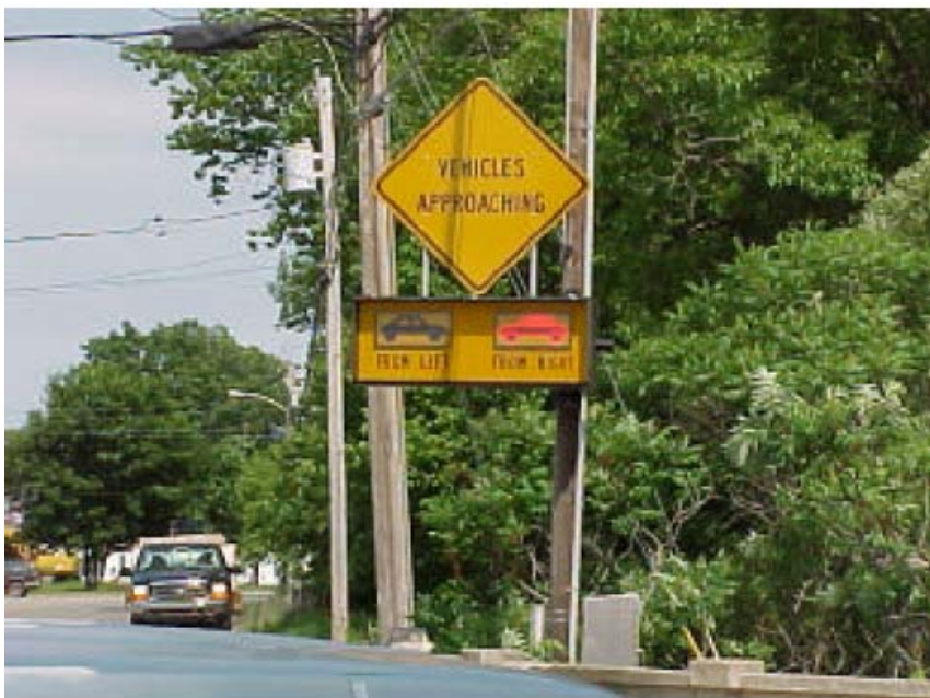
Figure 18 Vehicle Actuated Warning System (Norridgewock, Maine)
