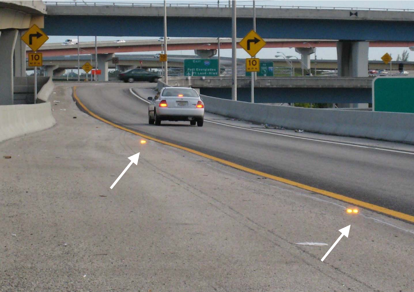
Vehicle Speed Actuated In-Pavement Lighting (Photo Source: Joseph Bansen)
