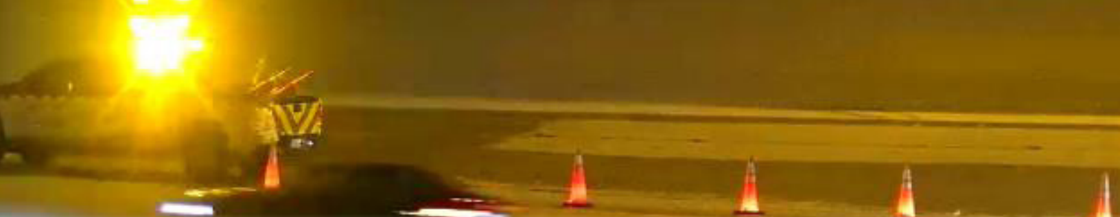
LED flare beneath cone illuminates the working zone of the road rangers (Photo: District 7)
