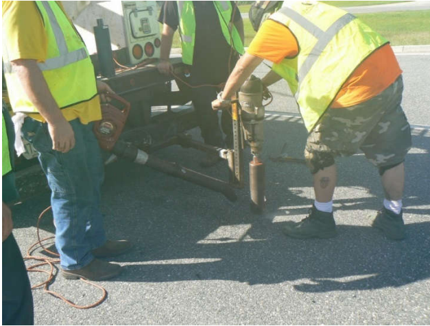
Figure 14. Core a hole into the pavement
