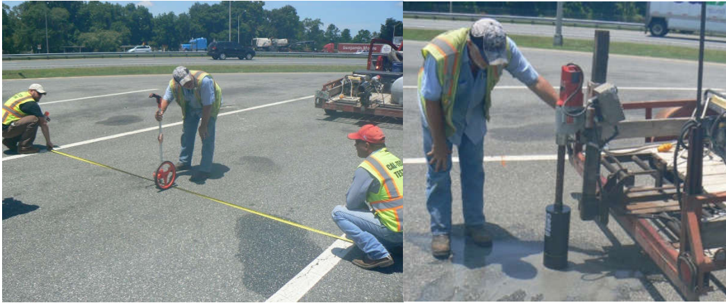
Figure 17. Mark the drilling point and drill a hole
