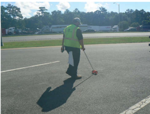
Figure 13. Find and mark the sensor location
