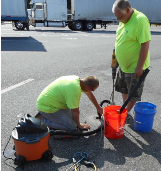
Figure 9. Vacuum the hole
