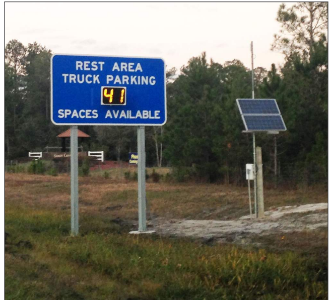
FIGURE 4. I-95 PILOT LOCATION DMS
