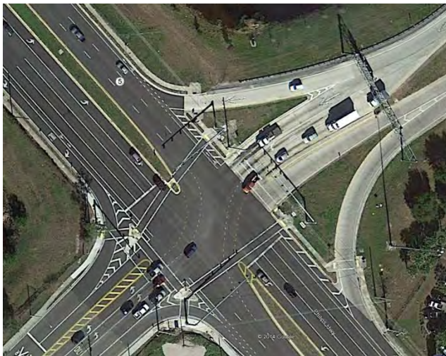
Narrow Ramp Median
