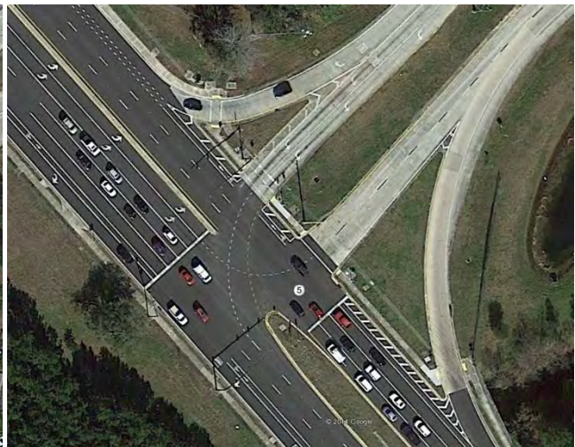
Wider Ramp Median
