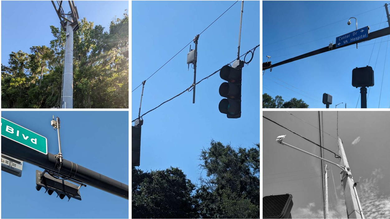
Figure 3-14: Examples of various roadside unit mounting scenarios
