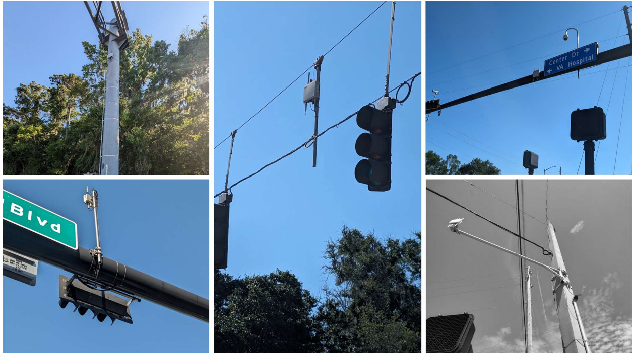
Figure 3-14: Examples of various roadside unit mounting scenarios
