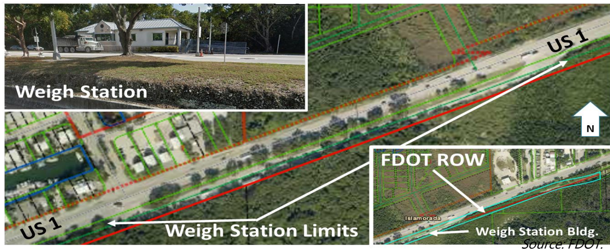
Figure 8-6 FDOT Weigh Station at Mile Marker 86
