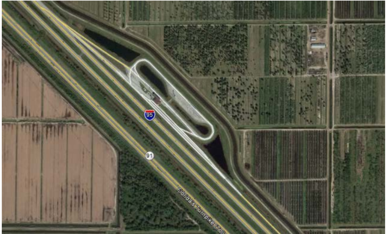
Figure A.26 Google Earth Aerial of Martin County Northbound Truck Comfort Station
