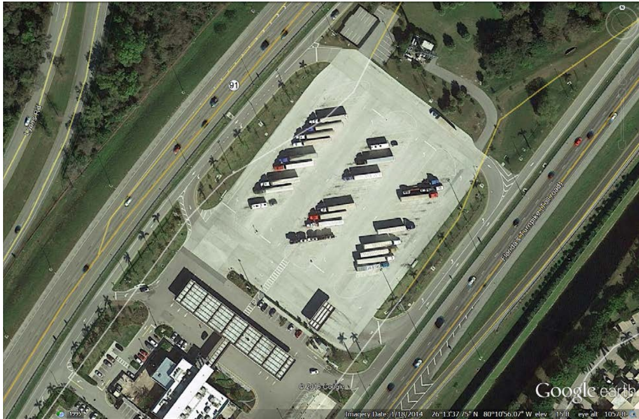
Figure A.42 Google Earth Aerial of Florida's Turnpike Plaza – Mile Post 65
