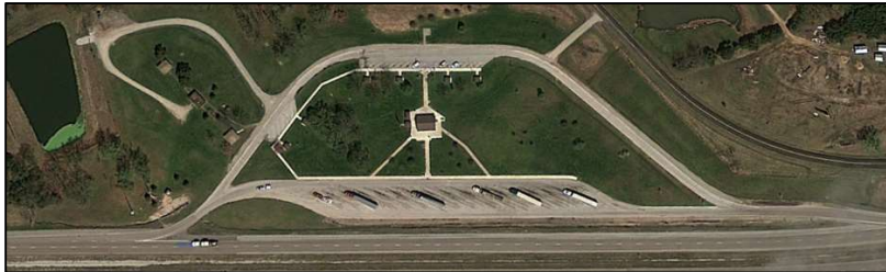
Figure 2-6a | Aerial of Interstate 70 (Danville, Missouri) Rest Area - Before Conversion
