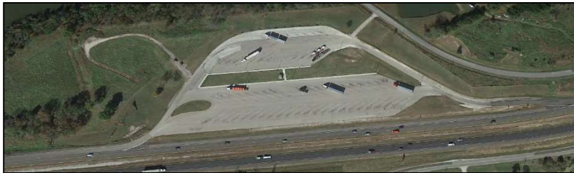
Figure 2-6b | Aerial of Interstate 70 (Danville, Missouri) Rest Area - After Conversion
