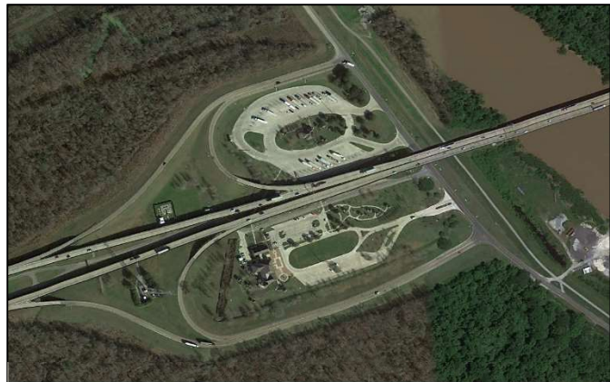
Figure 2-3 | LADOTD I-10 Rest Area
