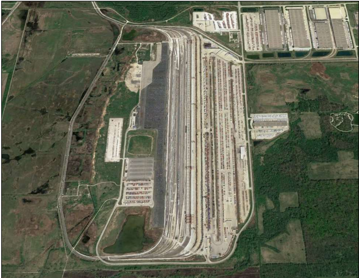
Figure 2-11 | Aerial of CenterPoint Intermodal Center
