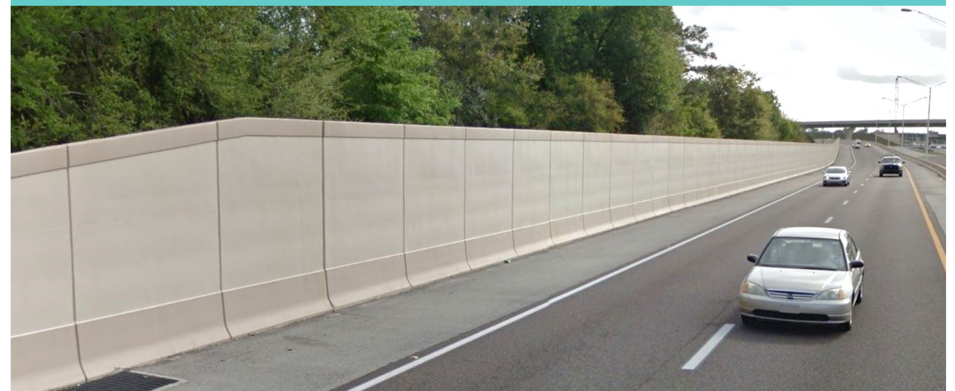
Example shoulder-mounted noise wall
