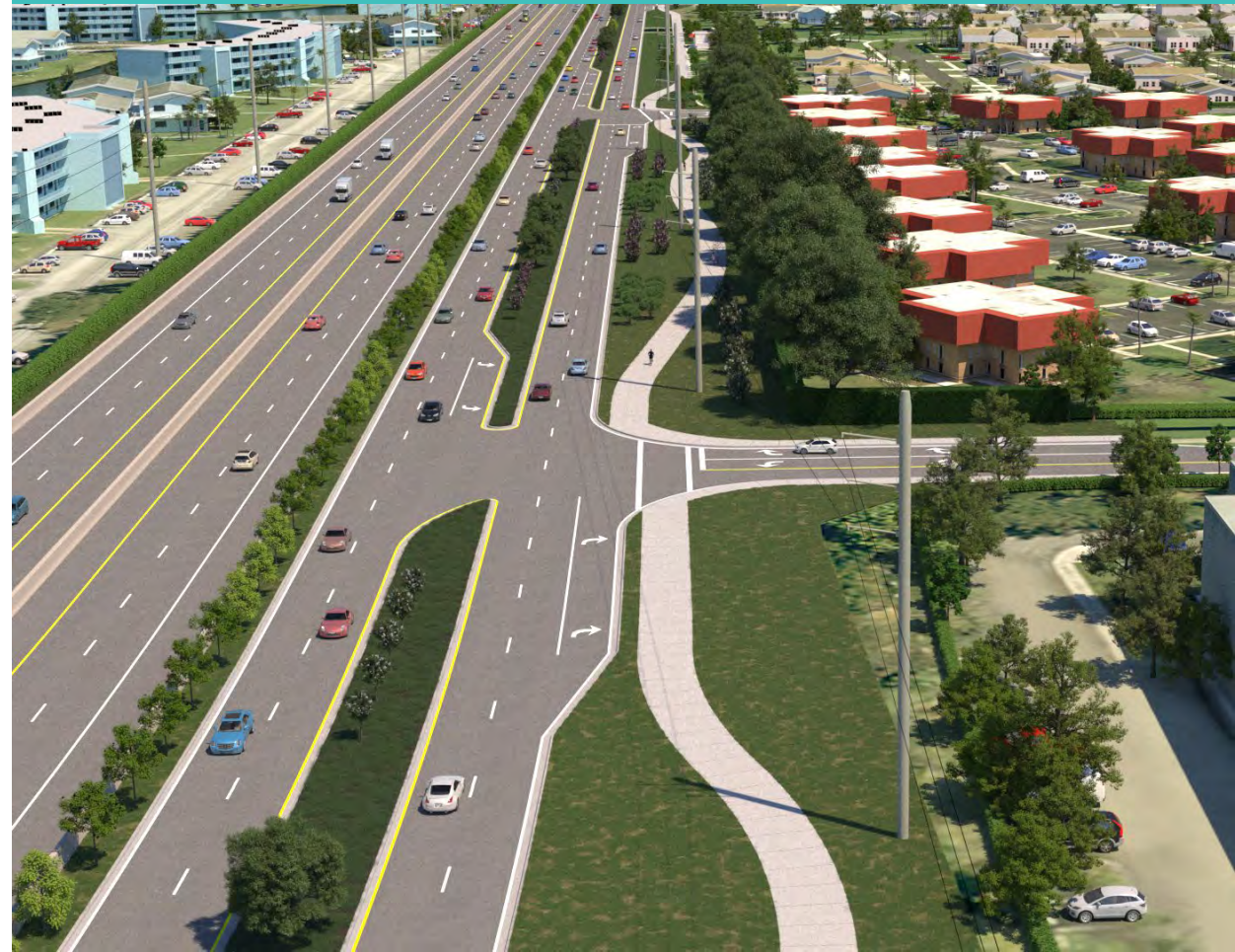
Without Powerline Road Ramps
