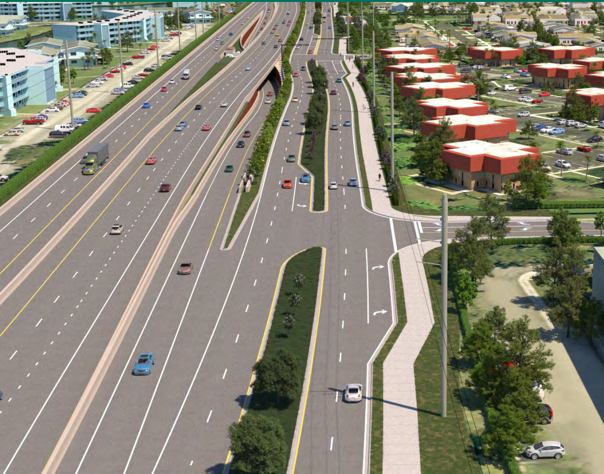
With Powerline Road Ramps
