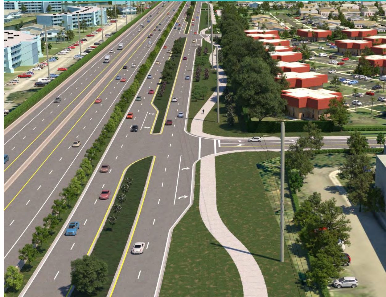
Without Powerline Road Ramps
