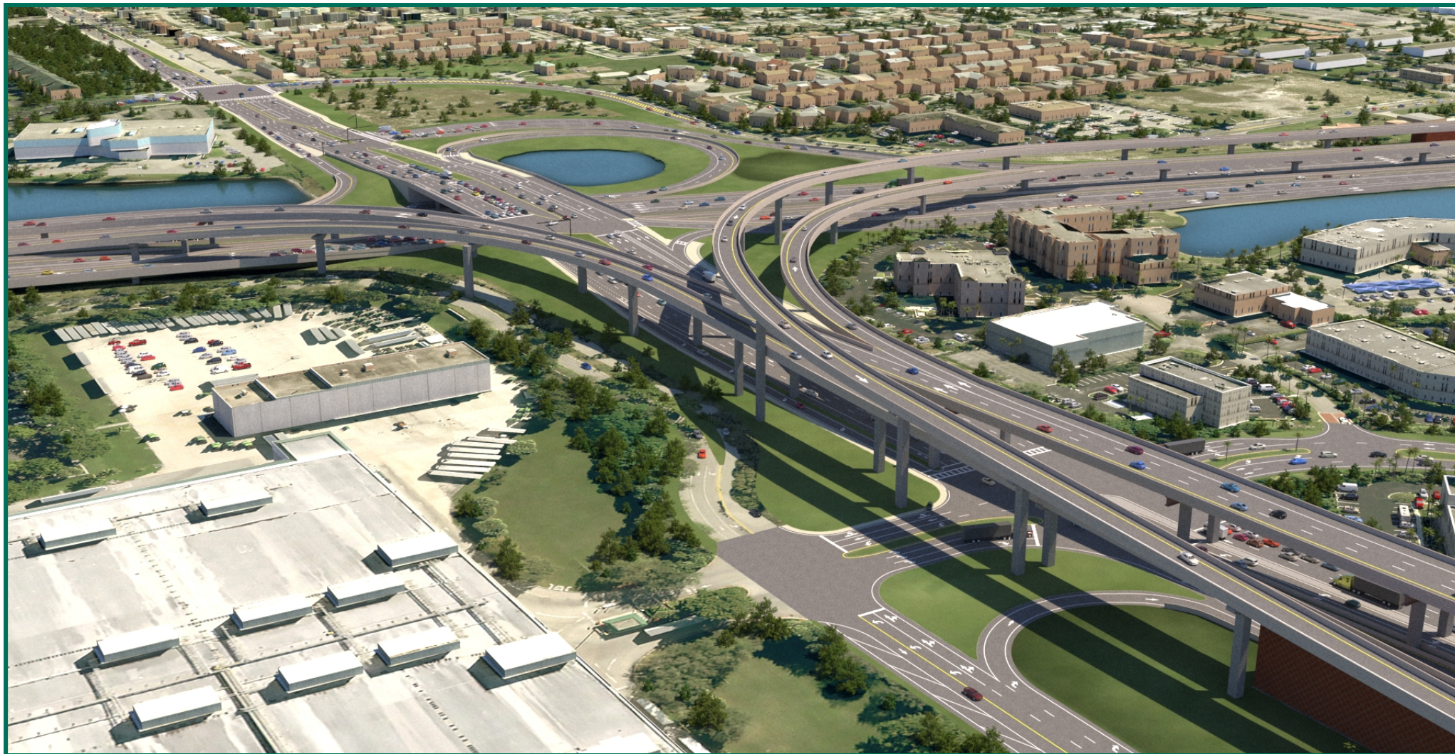
Camera 16: I-95 Interchange – Looking Southeast
