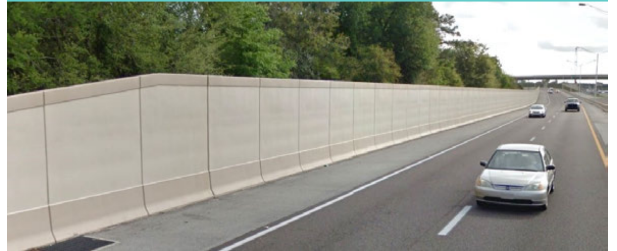
Example shoulder-mounted noise wall
