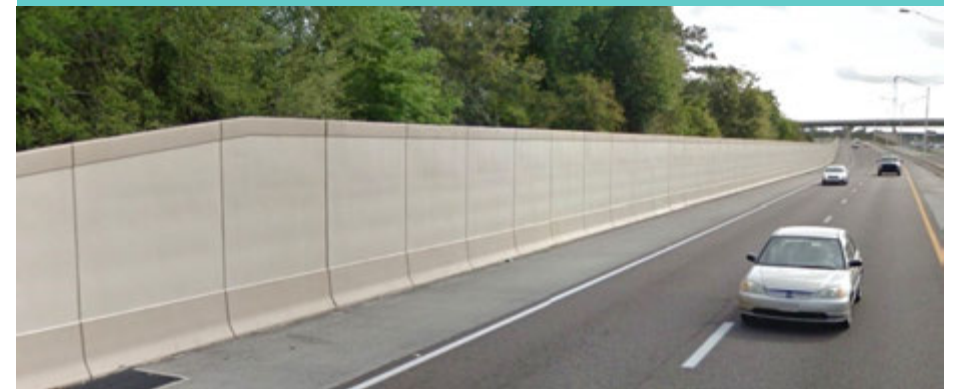
Example shoulder-mounted noise wall
