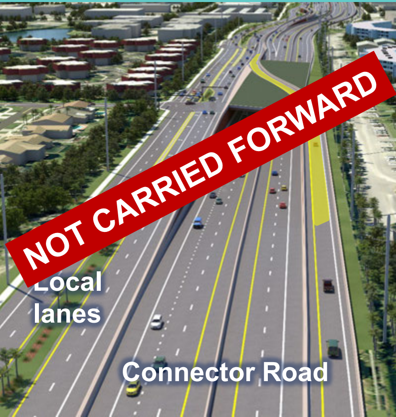
Depressed Eastbound and Westbound Managed Lanes
