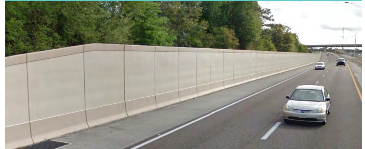
Example shoulder-mounted noise wall
