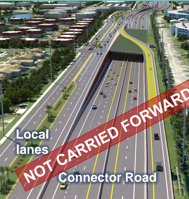
Depressed Eastbound and Westbound Managed Lanes
