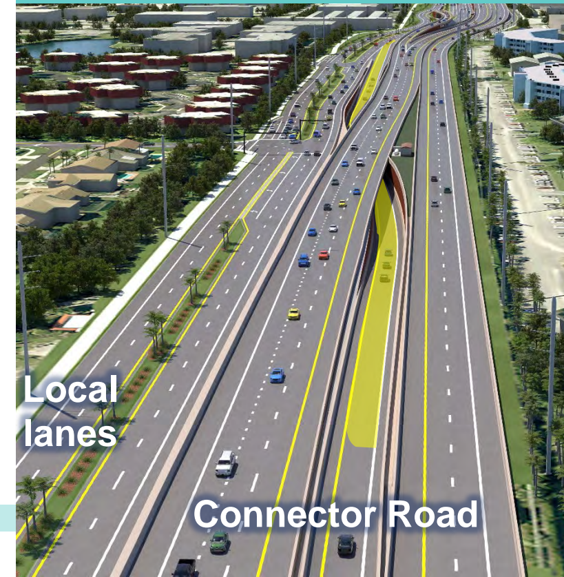
Depressed Westbound Exit Ramp
