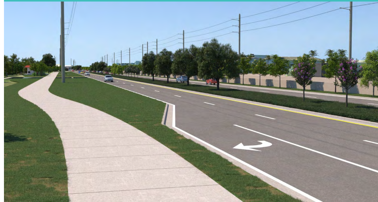
Without Powerline Road Ramps
