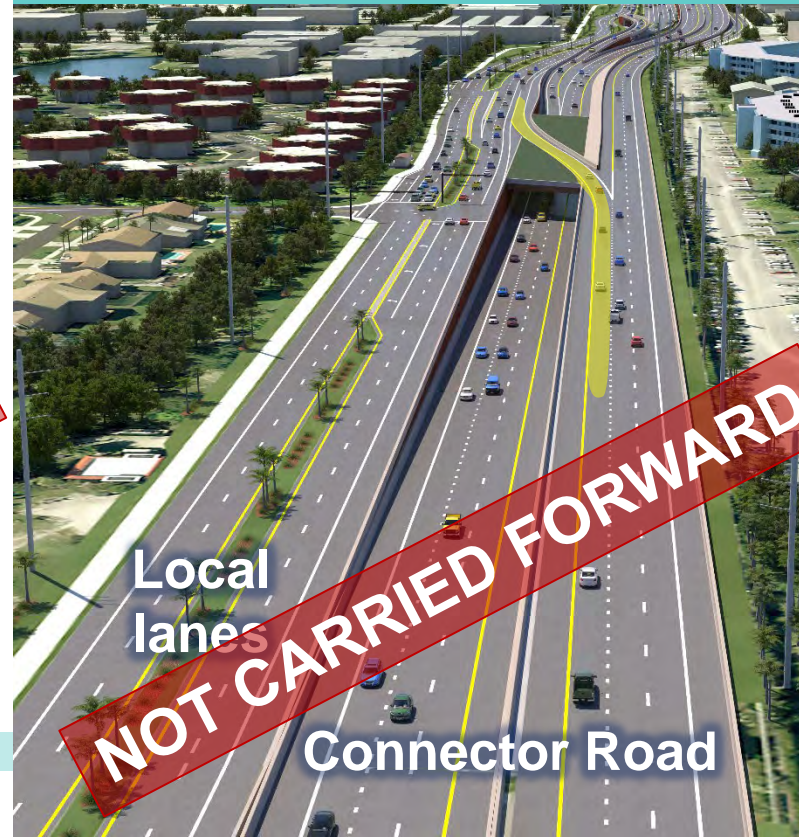
Depressed Eastbound Managed Lanes
