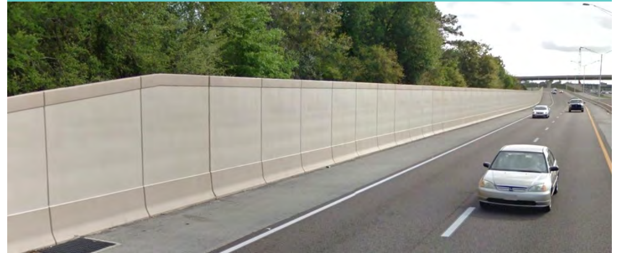
Example shoulder-mounted noise wall
