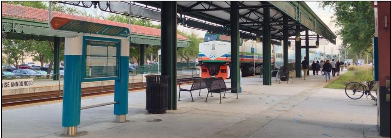
Figure 1 - 9: Deerfield Beach Station
