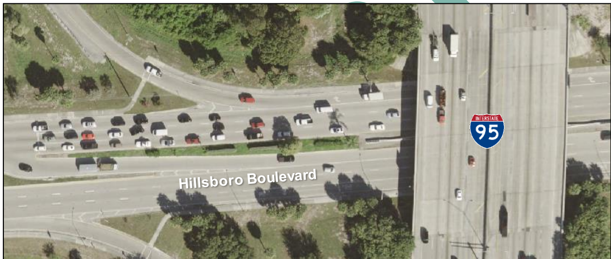
Figure 1 - 6: Existing Roadway Segment – Hillsboro Boulevard
