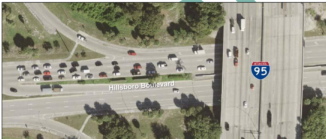
Figure 3 - 5: Existing Roadway Segment – Hillsboro Boulevard
