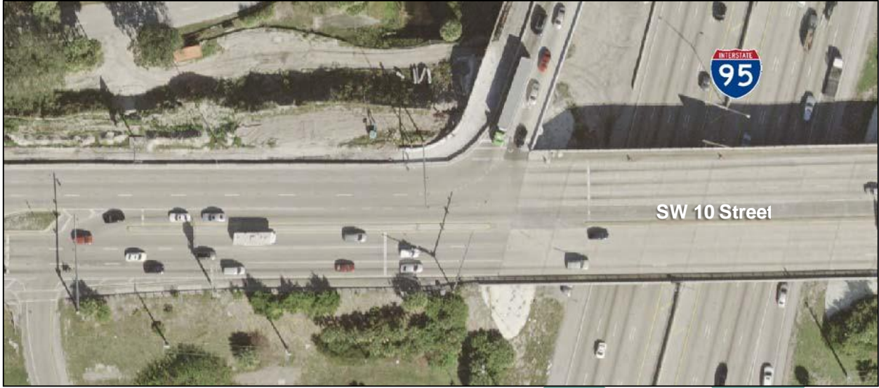
Figure 3 - 3: Existing Roadway Segment – SW 10 th Street
