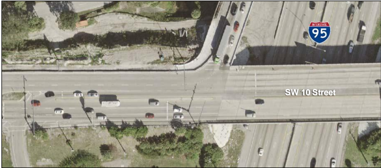
Figure 3 - 3: Existing Roadway Segment – SW 10 th Street
