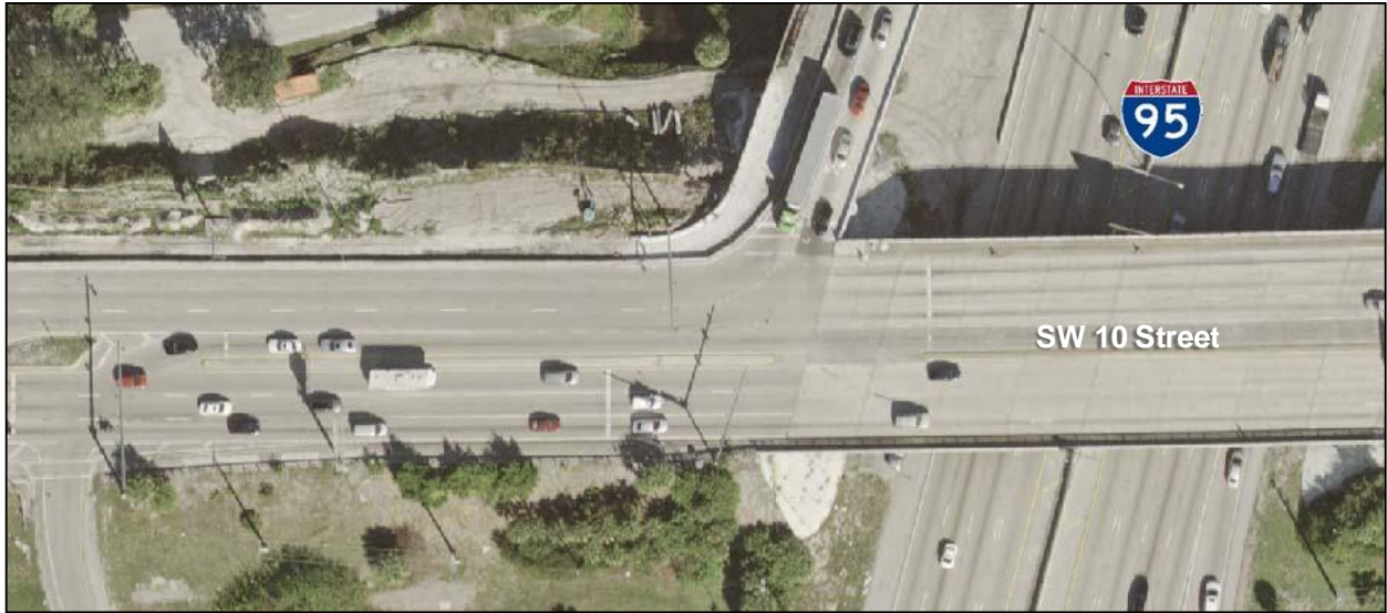
Figure 3 - 3: Existing Roadway Segment – SW 10 th Street
