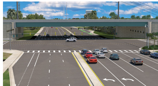
SW 10th Street Connector over Powerline Road: Looking North
