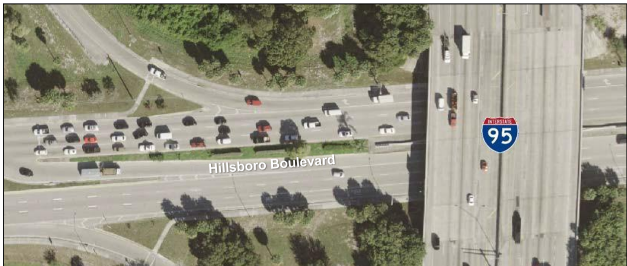
Figure 3 - 5: Existing Roadway Segment – Hillsboro Boulevard
