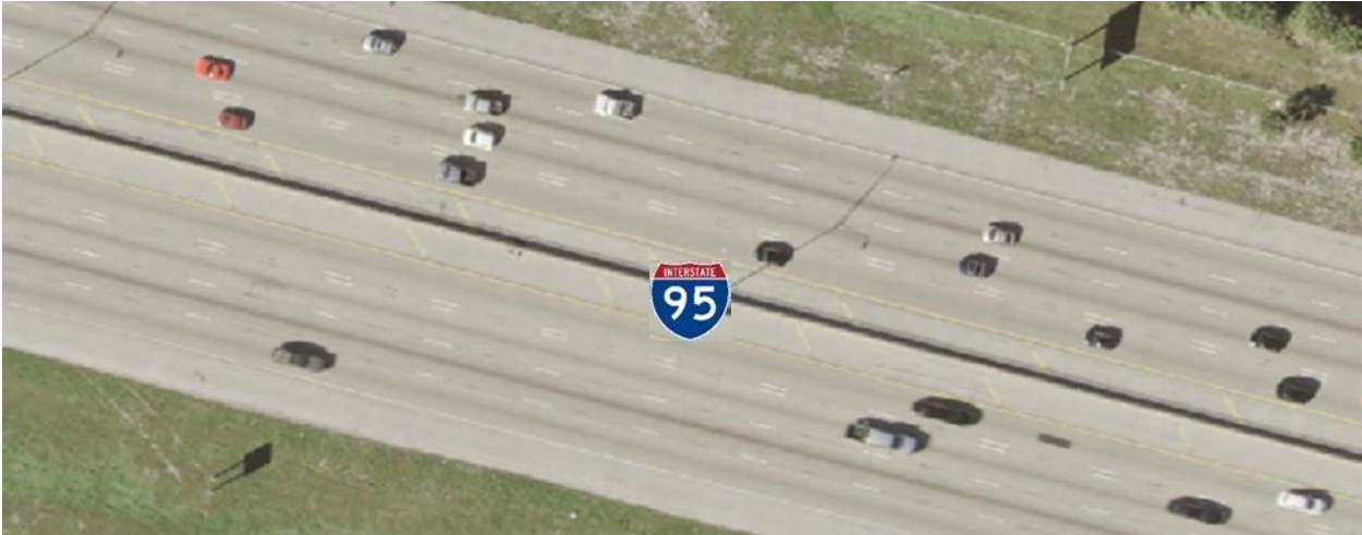
Figure 3 - 1: Existing Roadway Segment I-95 Corridor
