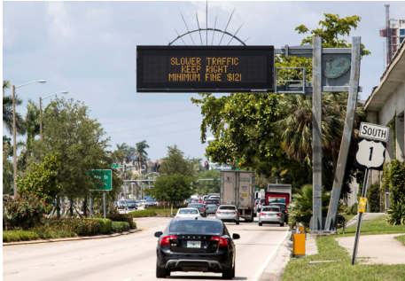
Overhead dynamic message signs providing real-time traveler information
