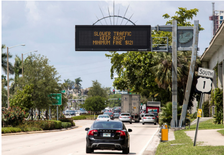
Overhead dynamic message signs providing real-time travel information
