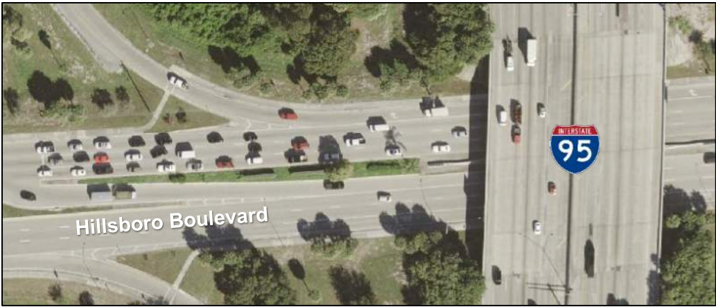
Figure 2-5 Existing Roadway Segment – Hillsboro Boulevard
