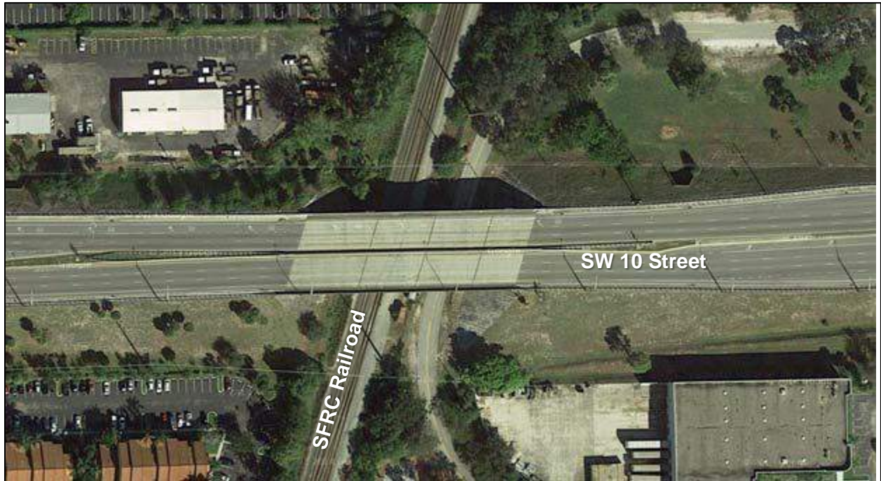
Figure 2-16 Bridges at SW 10 Street and SW 12 Avenue / SFRC Railroad Interchange (Bridge Nos. 860557 & 860553)
