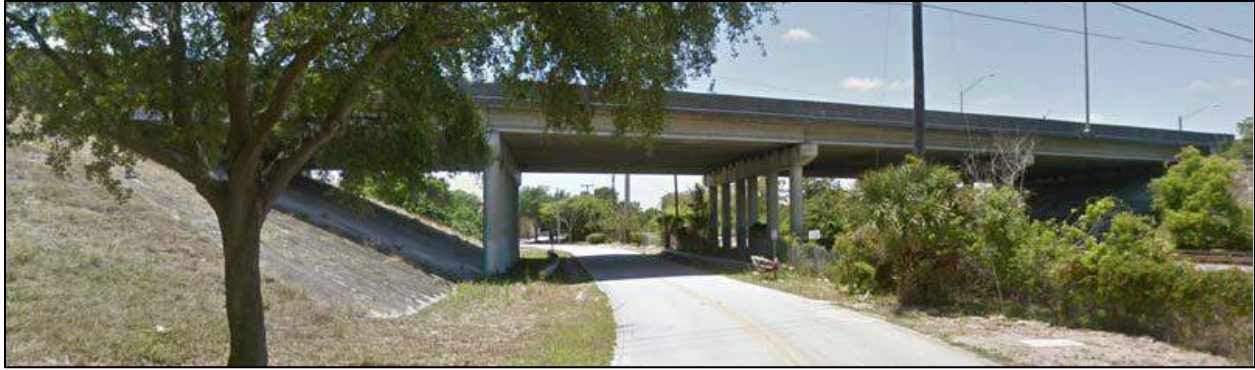
Figure 2-18 Bridge No. 860553 Looking South
