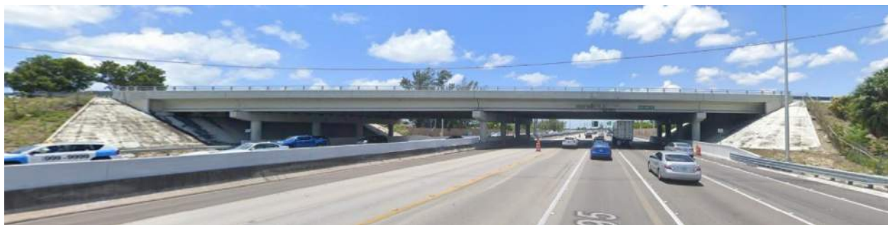
Figure 2-21 Bridge No. 860122 Looking South
