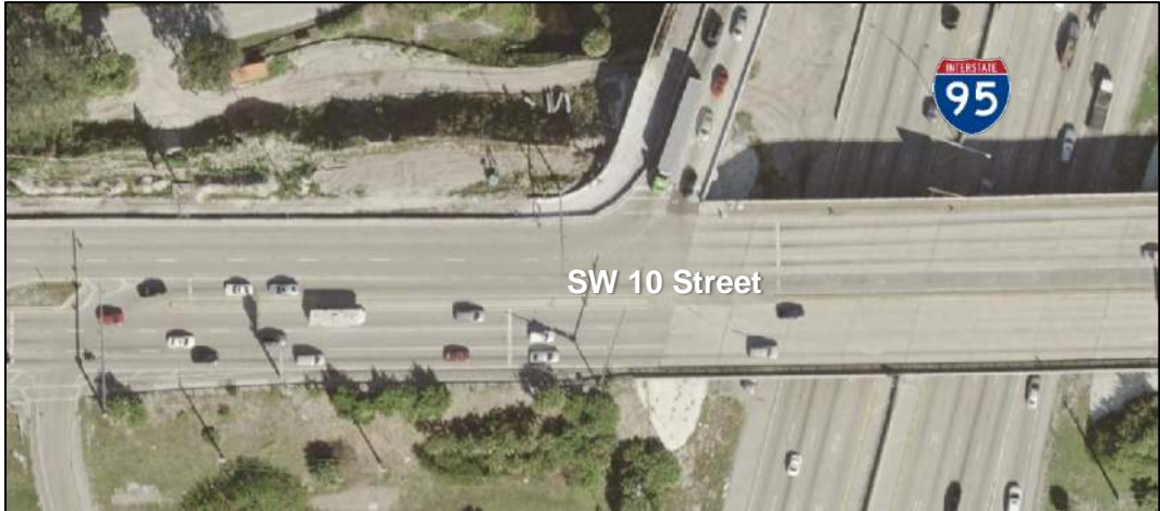
Figure 2-3 Existing Roadway Segment – SW 10 Street
