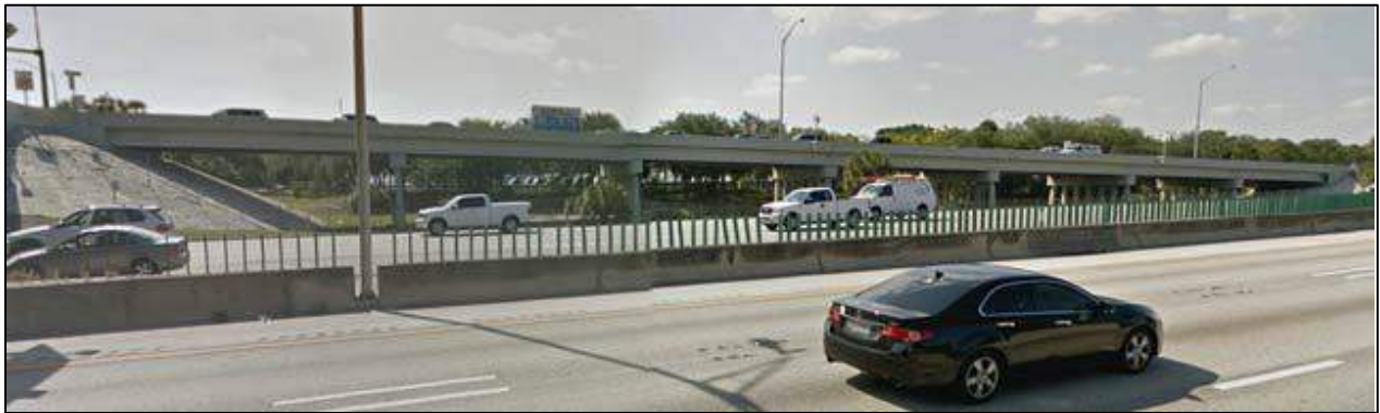
Figure 2-15 Bridge No. 860564 Looking West
