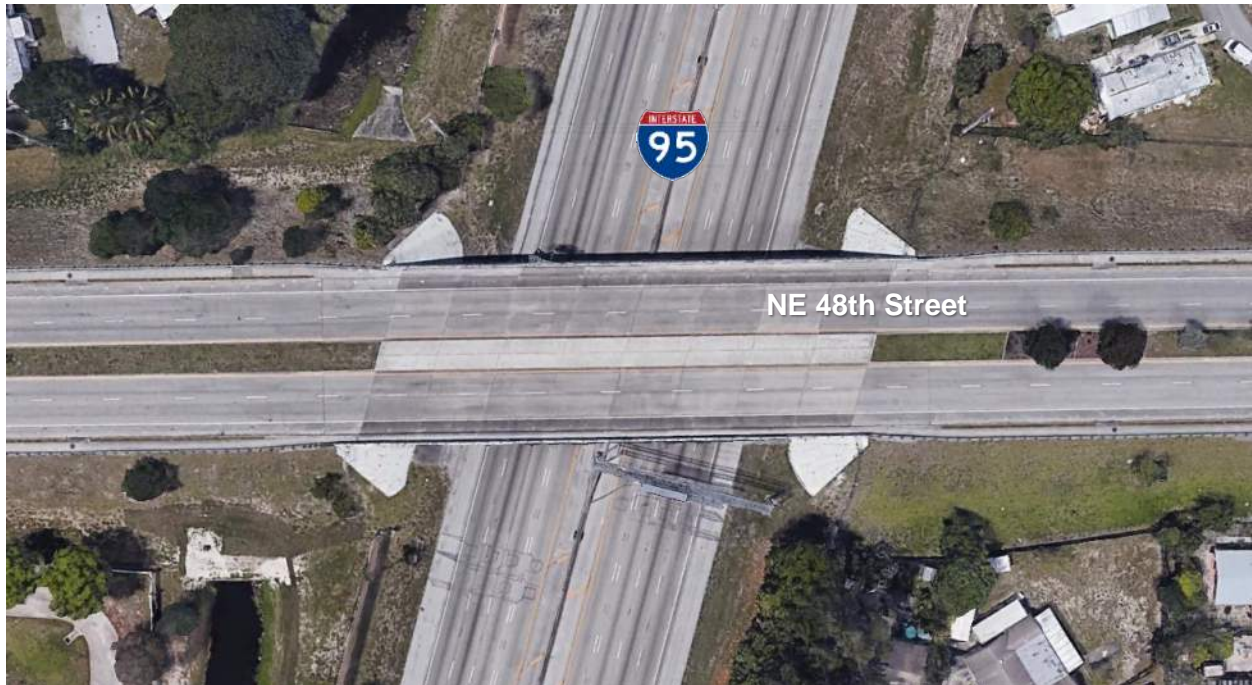
Figure 2-19 NE 48th Street and I-95 (Bridge No. 860122)
