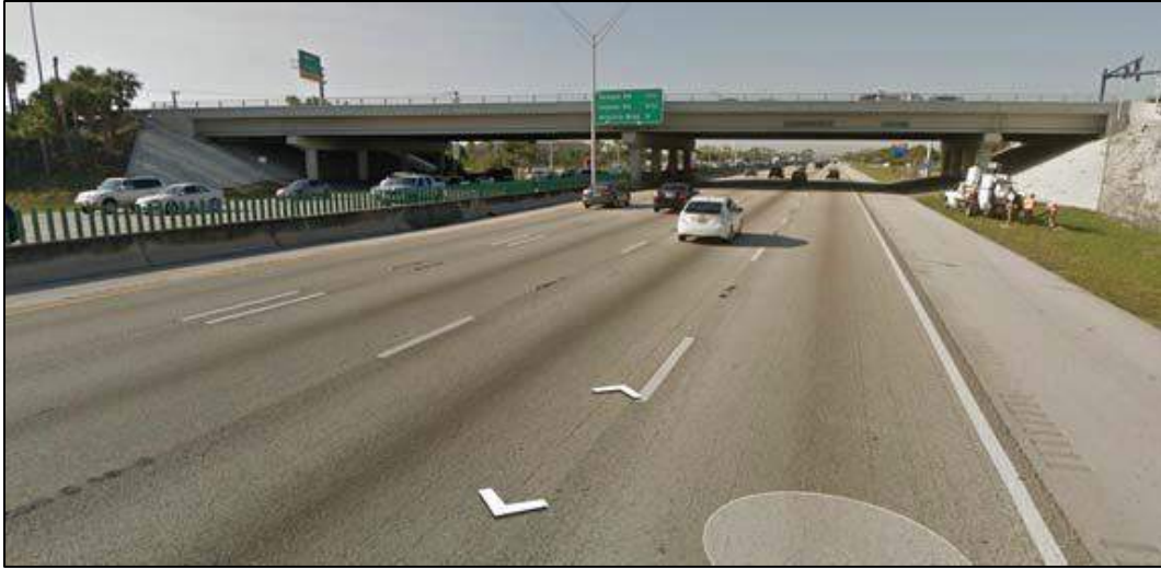
Figure 2-14 Bridge No. 860123 Looking South
