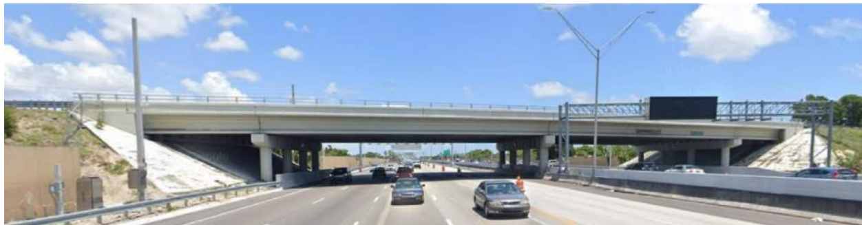
Figure 2-20 Bridge No. 860122 Looking North
