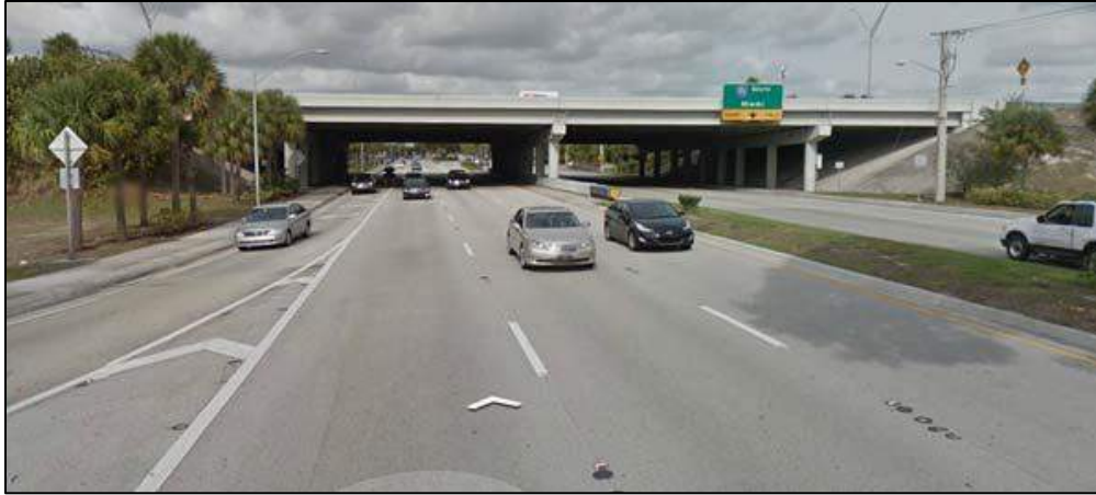
Figure 2-10 Bridge No. 860194 Looking West
