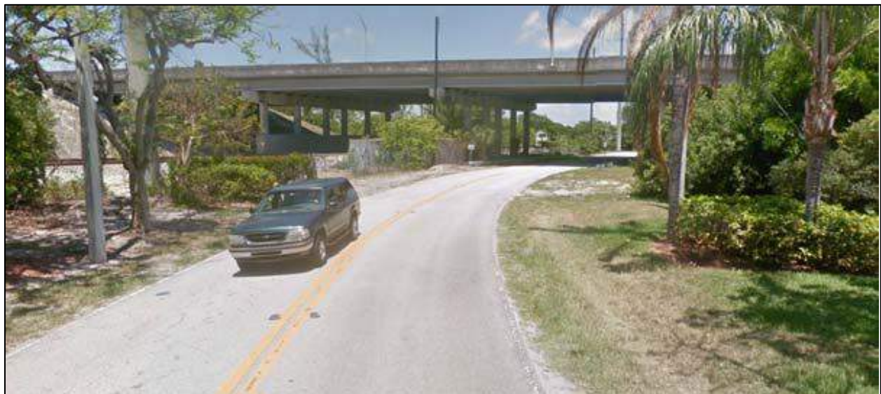
Figure 2-17 Bridge No. 860557 Looking North
