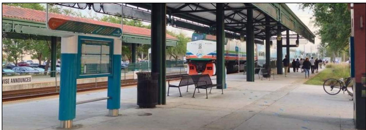
Figure 2-23 Deerfield Beach Station
