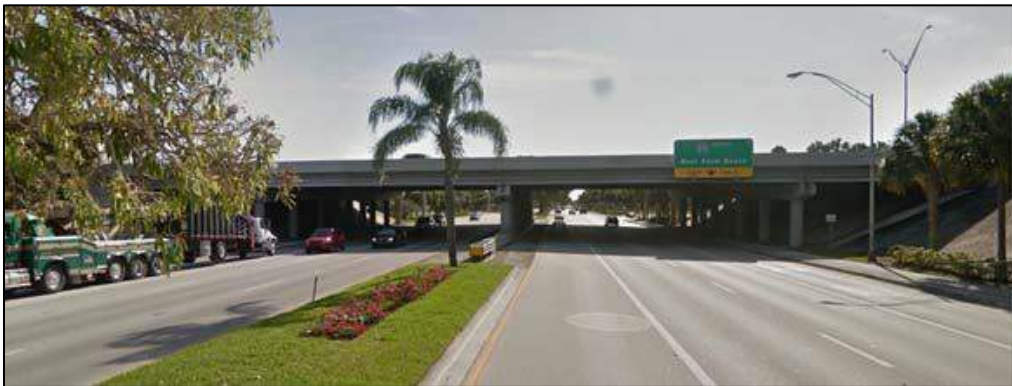
Figure 2-11 Bridge No. 860124 Looking East
