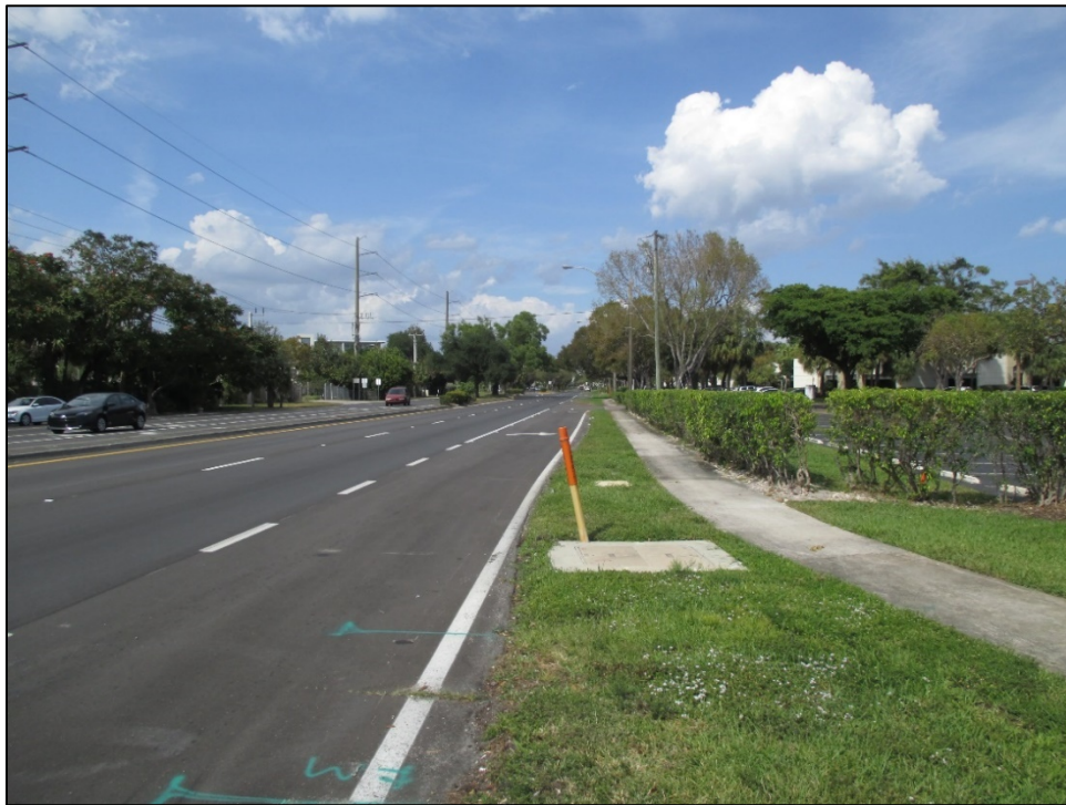
Figure 6-5 Buried Utilities, Sidewalk, and Landscaping along Military Trail, facing North
