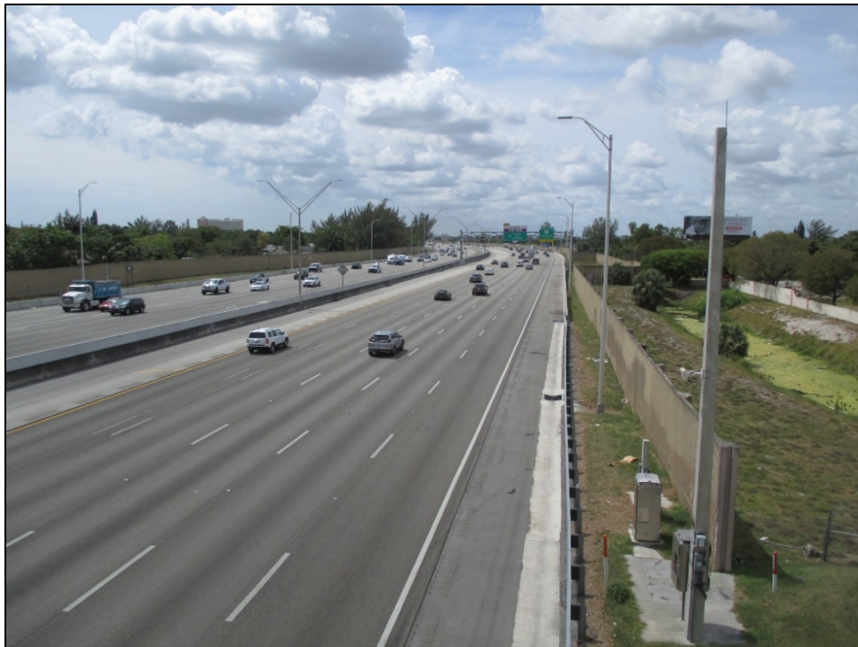
Figure 6-2 Buried Utilities along I-95 at 40th Street, facing South
