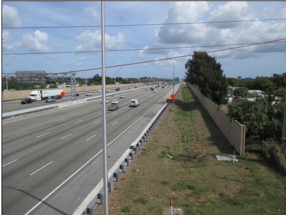
Figure 6-1 Buried Utilities and Ditch along I-95 at South End of Project Area, facing North
