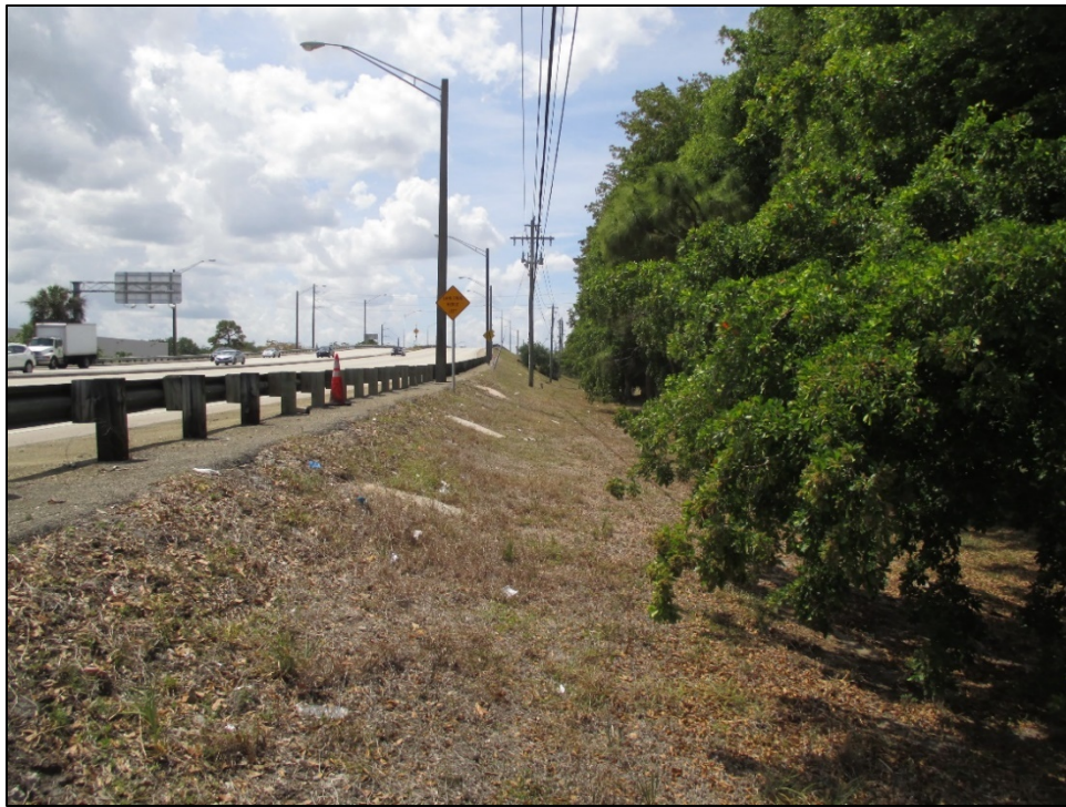
Figure 6-4 SW 10th Street at SW 12th Avenue, facing West
