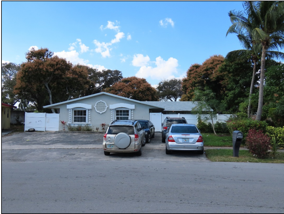
Figure 6-7 1201 SW 11th Avenue (8BD7743), c. 1973, considered National Register-ineligible, facing West
