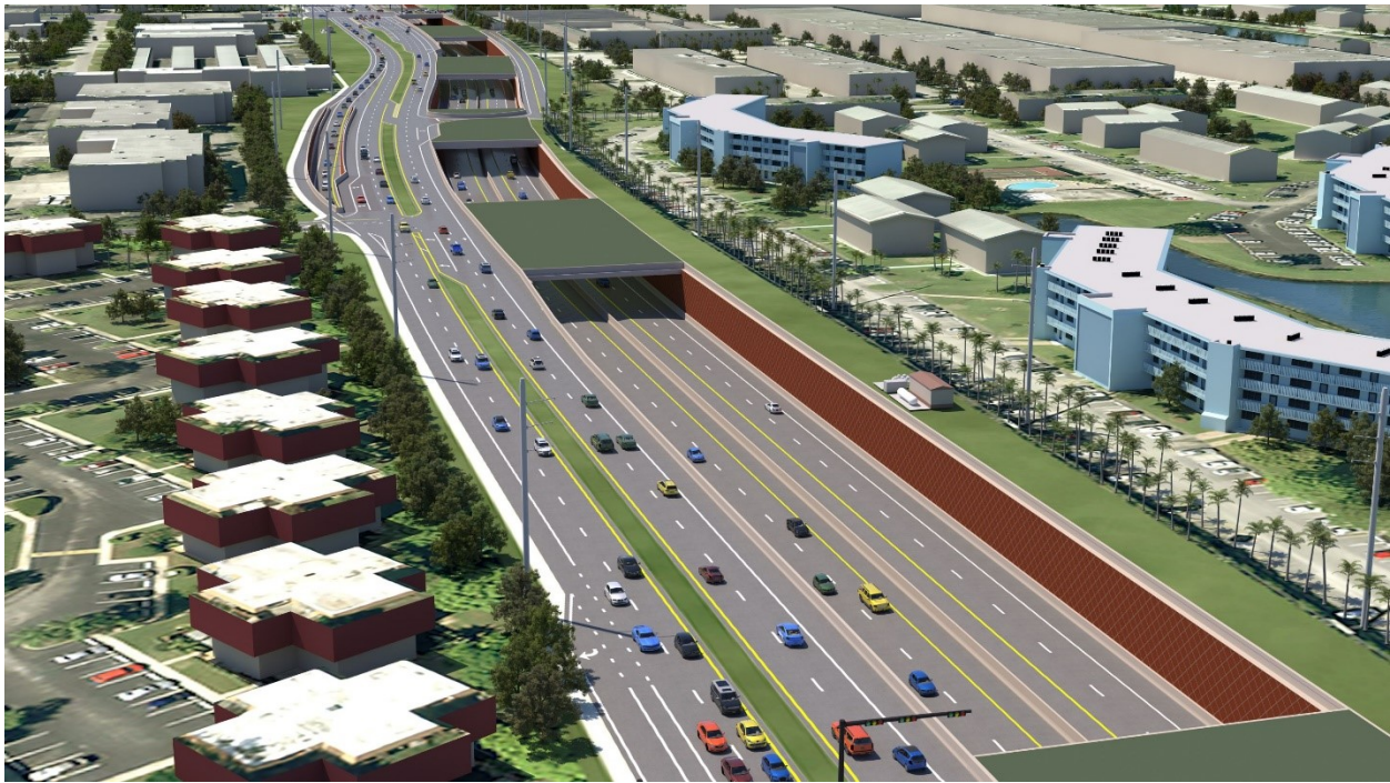
Figure 4.1.3: Full Depressed Alternative
