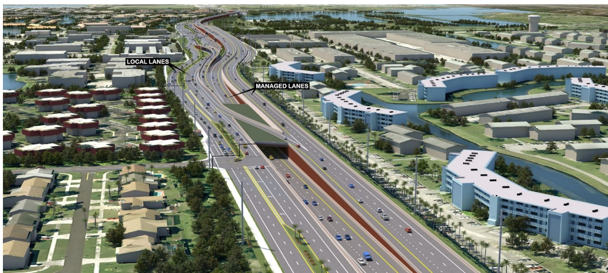
Figure 4.1.5: Partial Depressed – Depressed Eastbound Managed Lanes Alternative
