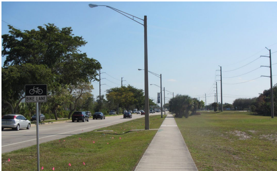
Figure 4-3: Existing Sidewalk and Bicycle Lane Photo on SW 10 th Street
