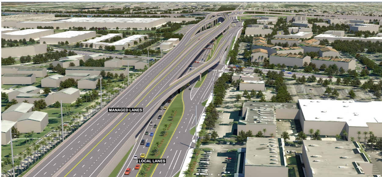
Figure 4.6.15: Depressed Westbound Exit Ramp Looking East
