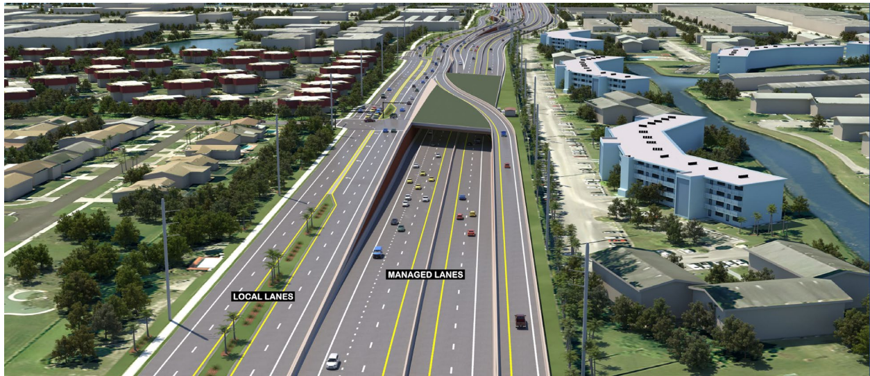
Figure 4.6.27: Depressed Eastbound & Westbound Managed Lanes Looking West
