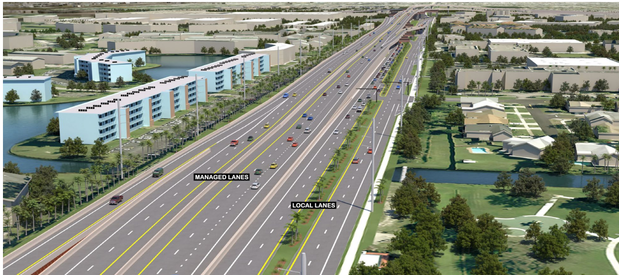
Figure 4.6.28: Depressed Eastbound & Westbound Managed Lanes Looking East
