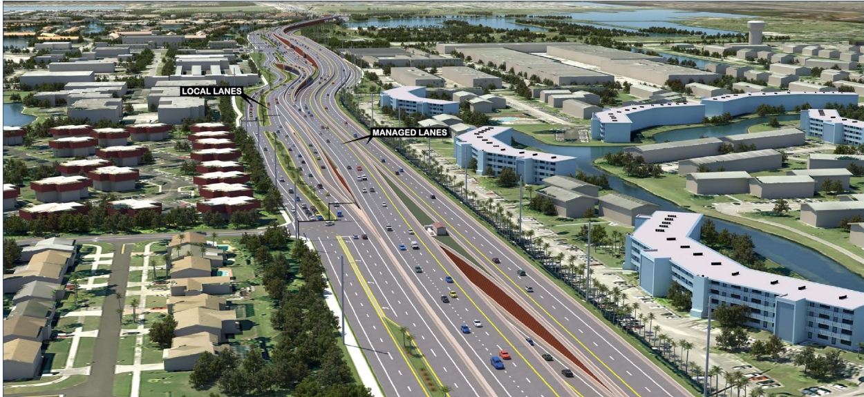
Figure 4.6.12: Depressed Westbound Exit Ramp Looking West
