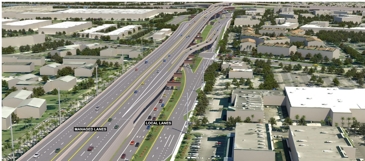
Figure 4.6.29: Depressed Eastbound & Westbound Managed Lanes Looking East
