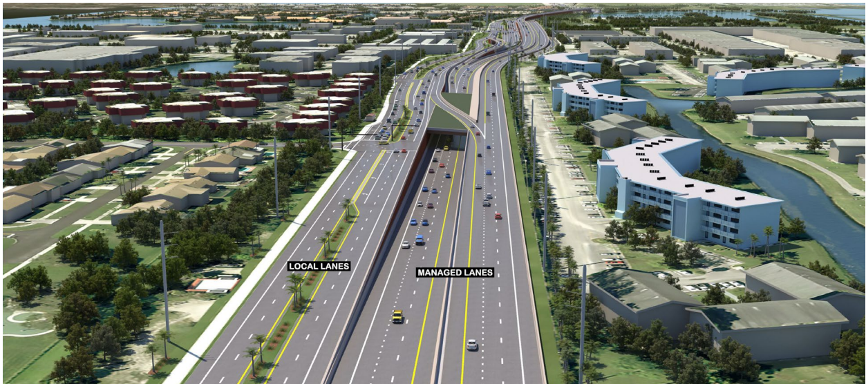
Figure 4.6.20: Depressed Eastbound Managed Lanes Looking West
