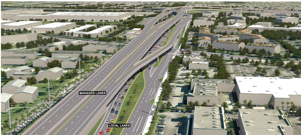
Figure 4.6.22: Depressed Eastbound Managed Lanes Looking East
