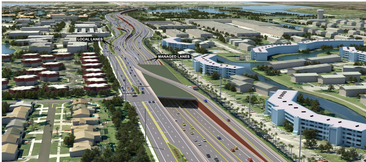
Figure 4.6.26: Depressed Eastbound & Westbound Managed Lanes Looking West
