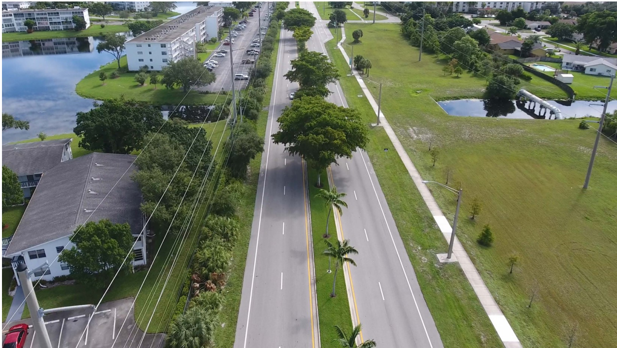
Figure 4.5.2: Existing Corridor Showing FP&L Transmission Lines (Looking East)
