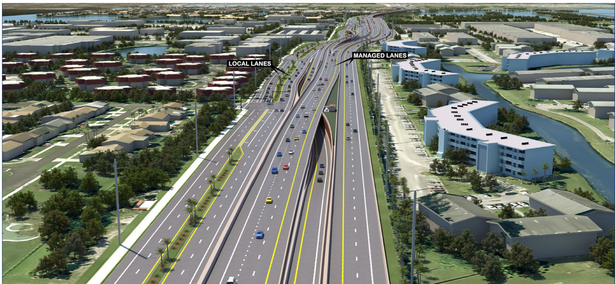
Figure 4.6.13: Depressed Westbound Exit Ramp Looking West
