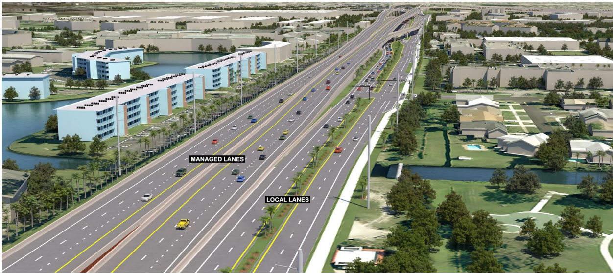
Figure 4.6.21: Depressed Eastbound Managed Lanes Looking East
