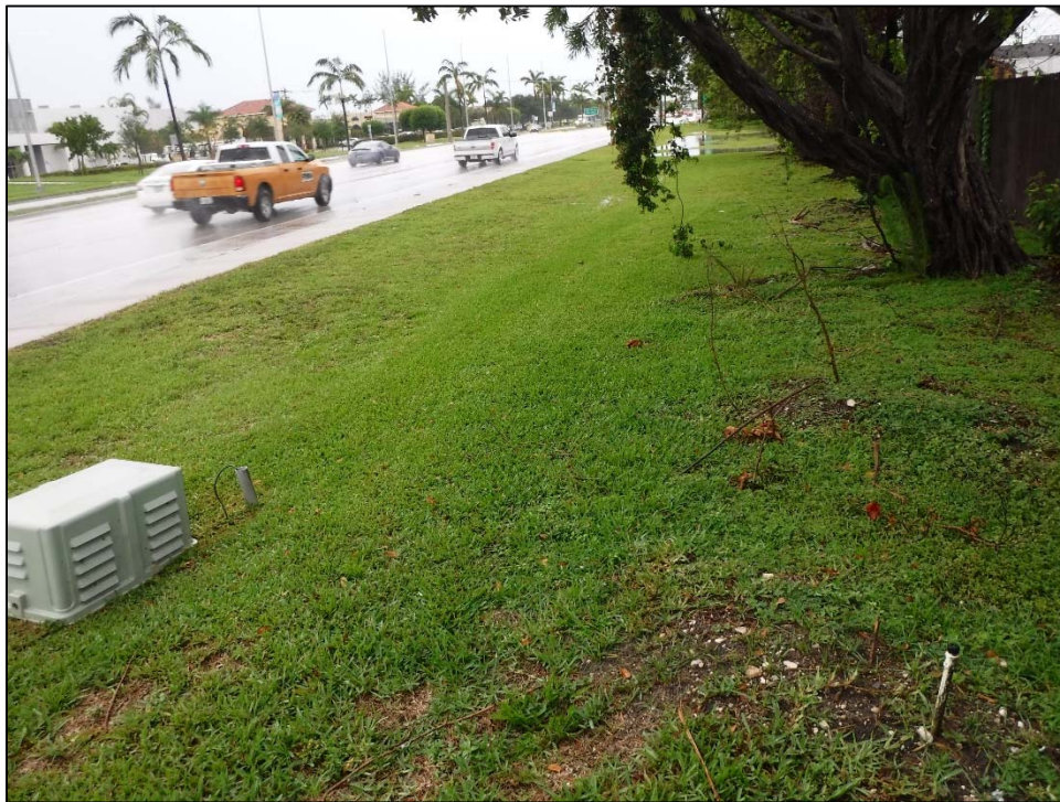
Figure 9.1.3: Drainage Ditches and Buried Utilities on Powerline Road, Facing North
