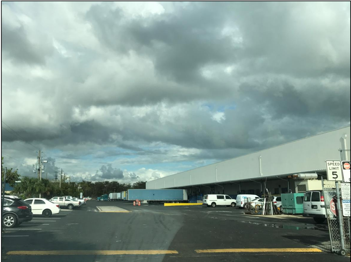
Site 20 – Rexall Sundown, 1111 SW 30 th Avenue, one underground storage tank
