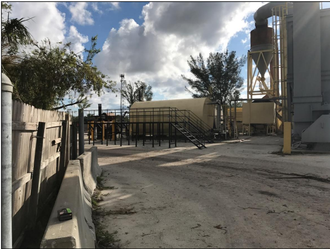
Site 22 – Hardrives Asphalt Co, 1200 S Powerline Road, ASTs were confirmed
