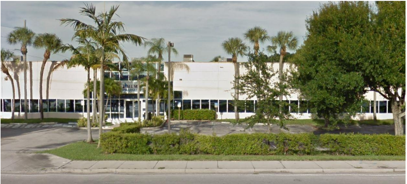
Folio: 484210020040 Description: Med-Care Pharmacy Building and Parking
