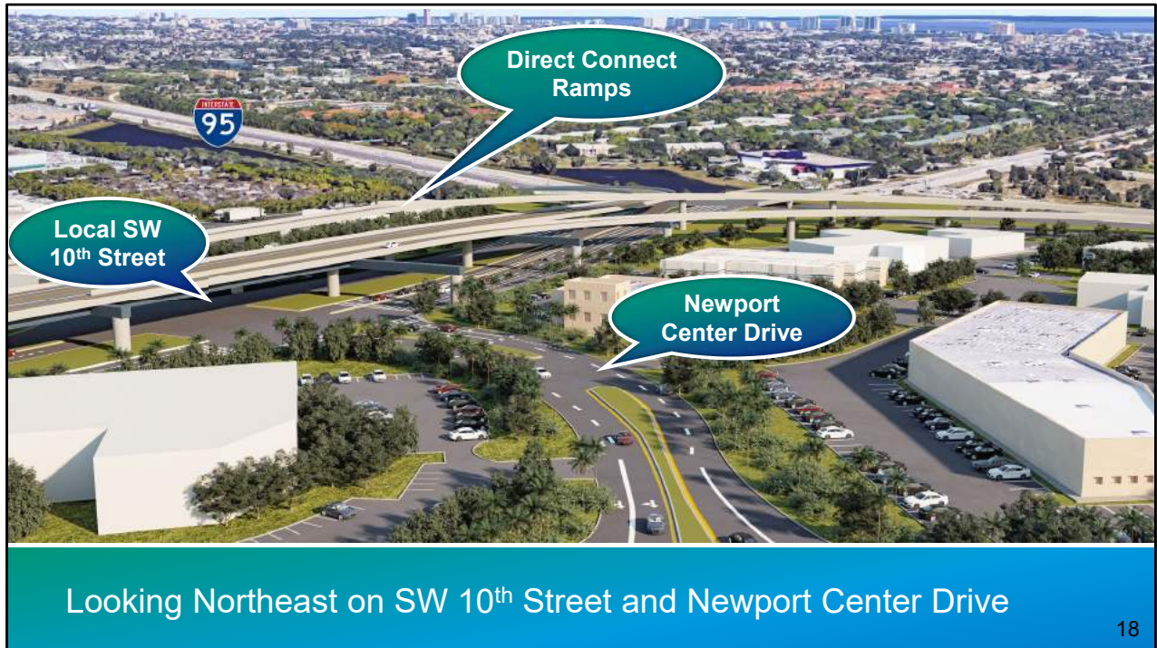
Rendering looking NE at SW 10 th Street and Newport Center Drive showing the local SW 10 th Street as well as the managed lanes and direct connect ramps.
