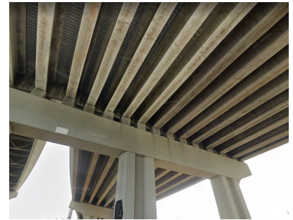
The I-beam is widely used in bridge and overpass construction because it allows for longer spans at lower weight.
