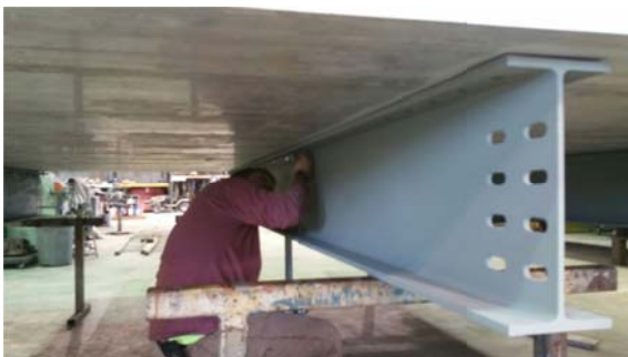
Figure 20 – Bolt Installation
