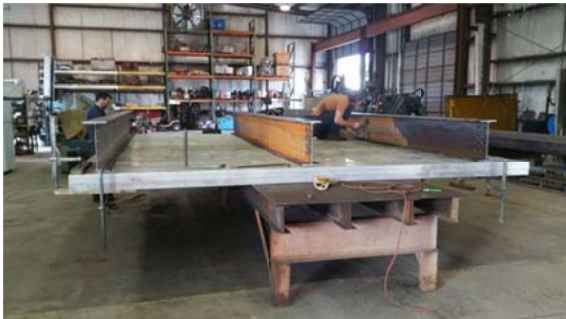
Figure 18 – Transferring Holes to Deck Panel
