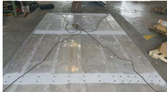
Figure 19 – Sand Blasting Panel Bottom
