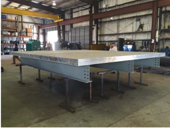
Figure 22 – Completed Deck Unit
