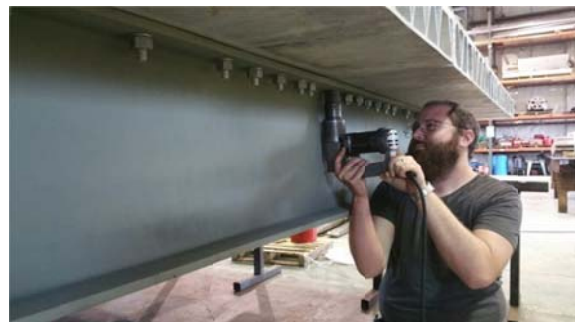
Figure 21 – TC Bolt Tightening
