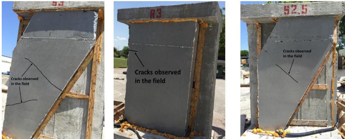
Figure 5-4: Cracks in pourback specimens
