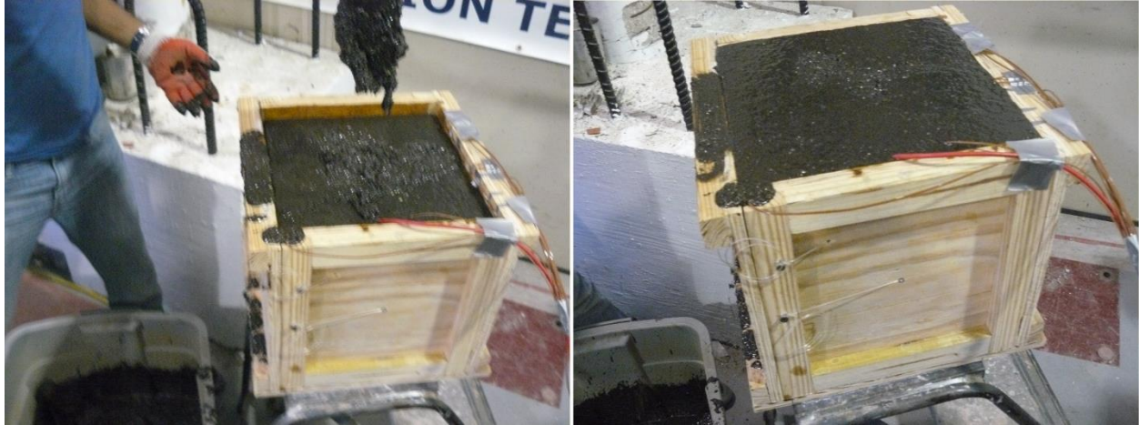
Figure A-9: The E3-HP epoxy grout was placed in one lift
