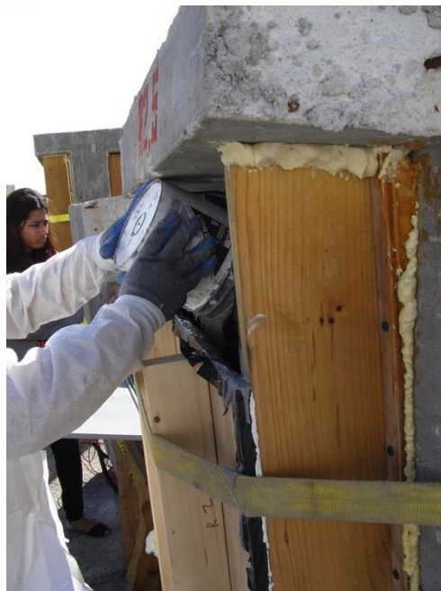
Figure 4-6: Mixing and casting of epoxy pourback
