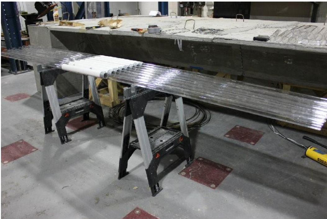
Figure D2. Ducts for Post-tensioning
