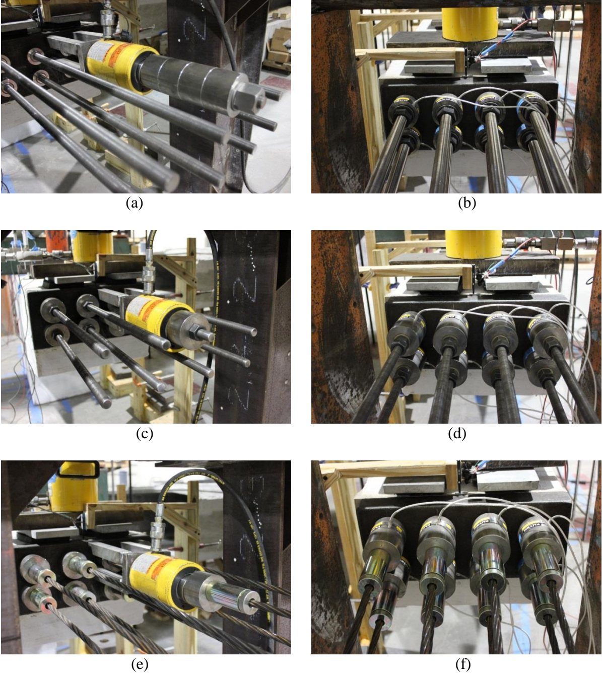
Figure 3.5 Post-Tensioning System: (a) Live End for CFCC, (b) Dead End for CFCC, (c) Live End for EC6, (d) Dead End for EC6, (e) Live End for Steel, and (f) Dead End for Steel
