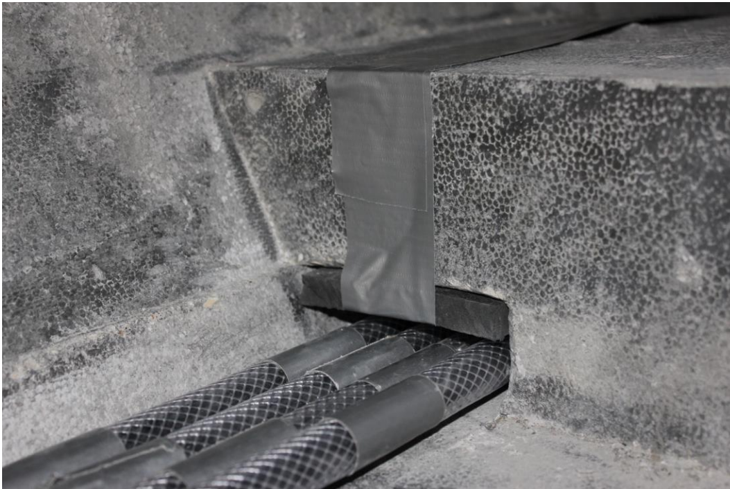
Figure A10. Protecting the Post-Tensioning Cables at Deviator Block
