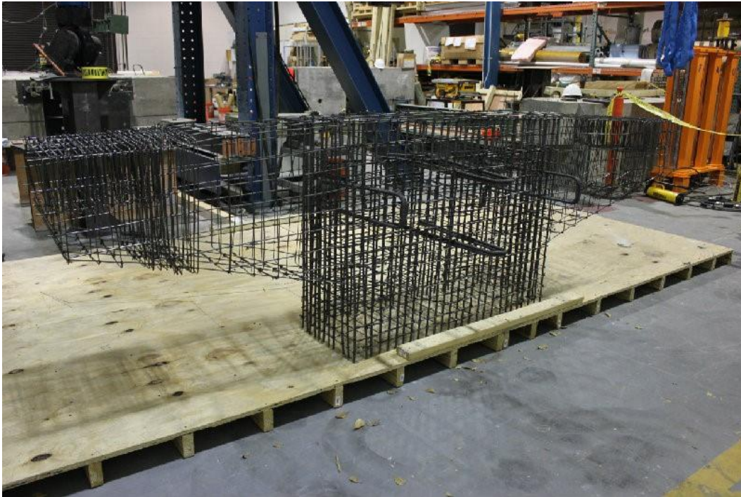
Figure D3. Reinforcement Cage
