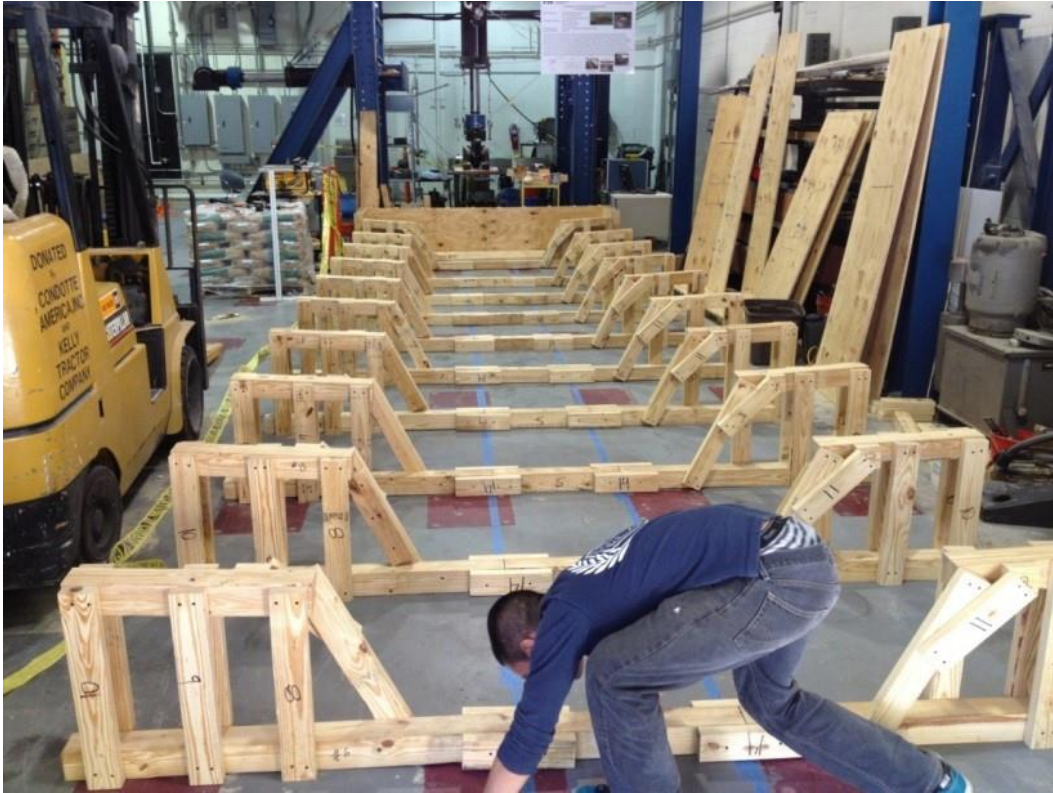
Figure A1. Formwork Framing
