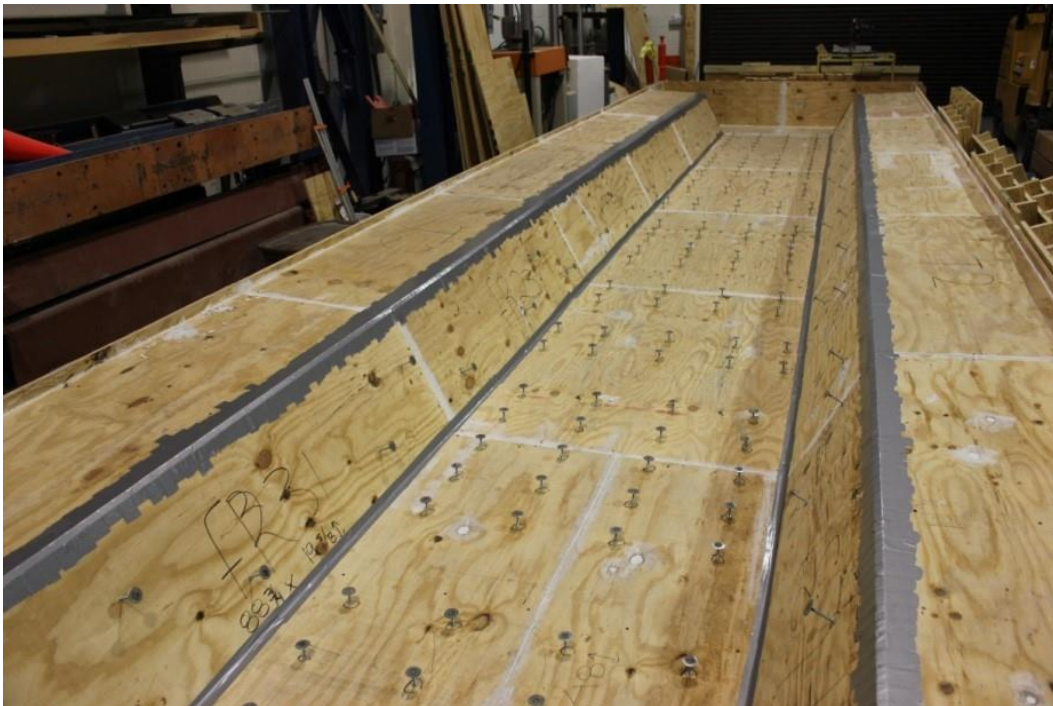
Figure A2. Formwork Base
