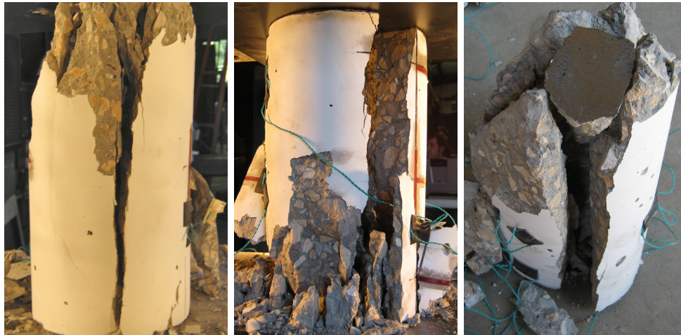
(a) Crack parallel to cylinder axis (b) Vertical cleavage (c) Small cone on top end
