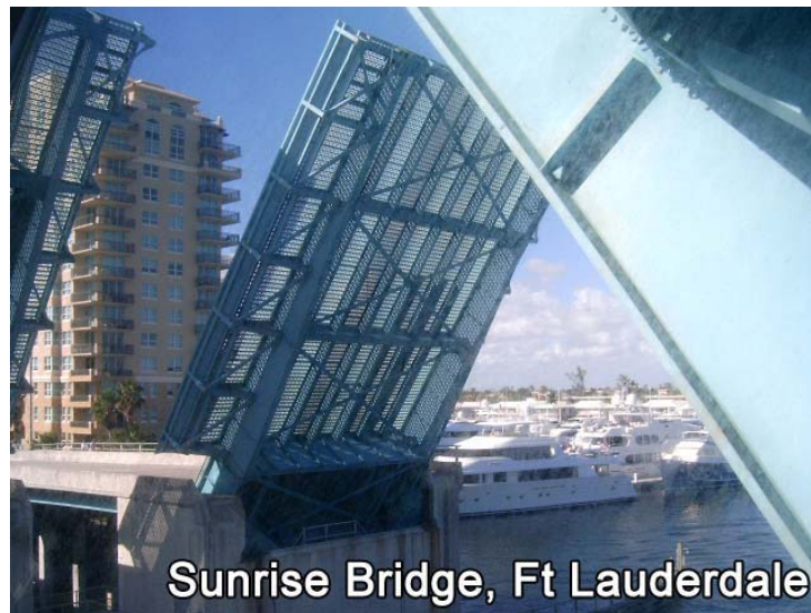
Figure 30: Structural components of Sunrise Boulevard Bridge
