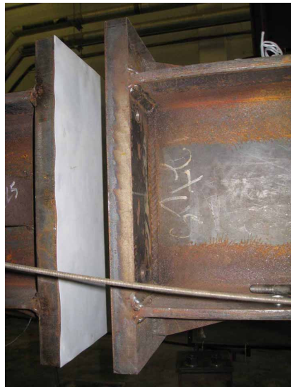
Figure 7-22. Teflon sheet placed between flange plates
