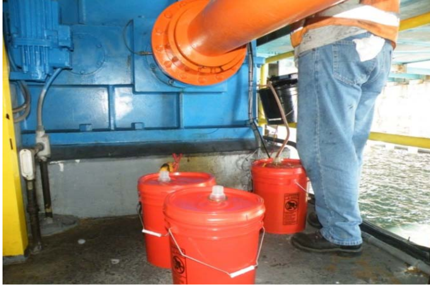
Figure 131: Removal of the Oil from the Gearbox
