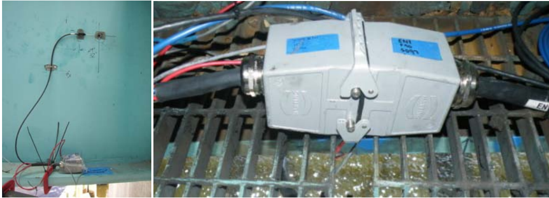
Figure 30: Sensor Group Installation (Left) and Cable Connected Installation (Right)
