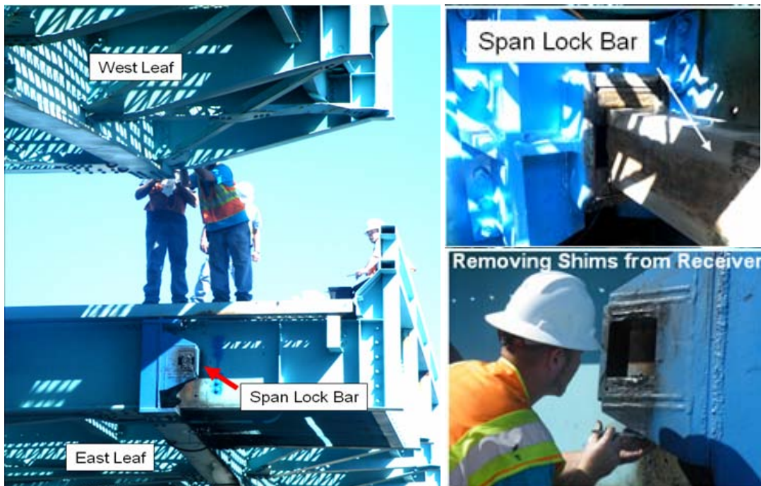
Figure 130: FDOT Contractors Removing Some of the Shims from the SL
