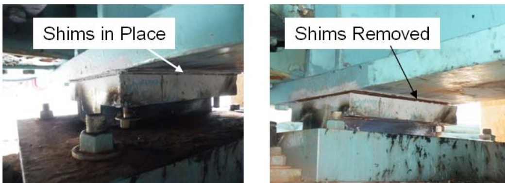
Figure 127: LLS with Shims and Without Shims
