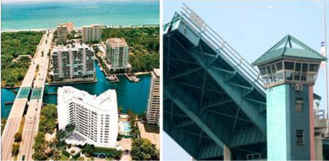
Figure 1: Sunrise Bridge in Ft. Lauderdale, Florida
