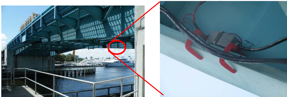
Figure 31: Installed Connector Secure on the Bottom Flange of the Main Girder
