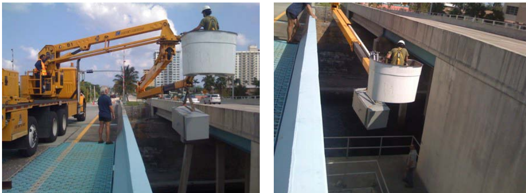
Figure 56: Moving the Cabinets with Snooper Truck
