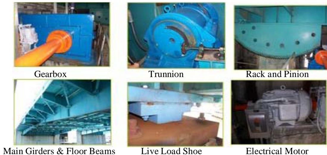
Figure 11: Some of the Monitored Bridge Components
