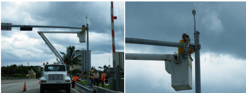
Figure 58: Installation of the Weather Station and Traffic Camera
