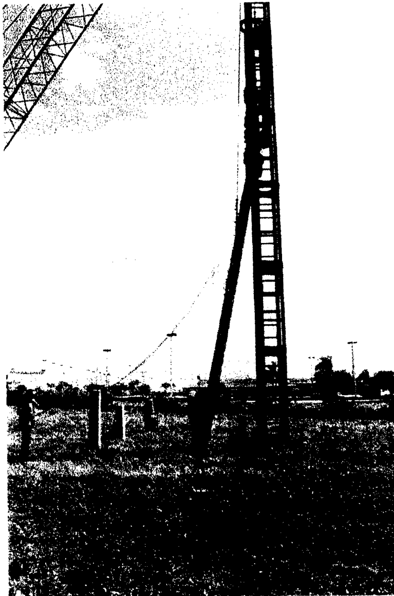
Figure 11.4 Positioning of CFRP pretensioned pile
