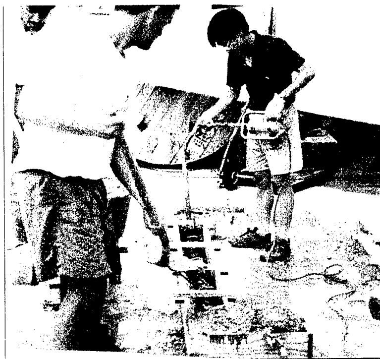
Fig. 5.6 Preparing the formwork and reinforcement
