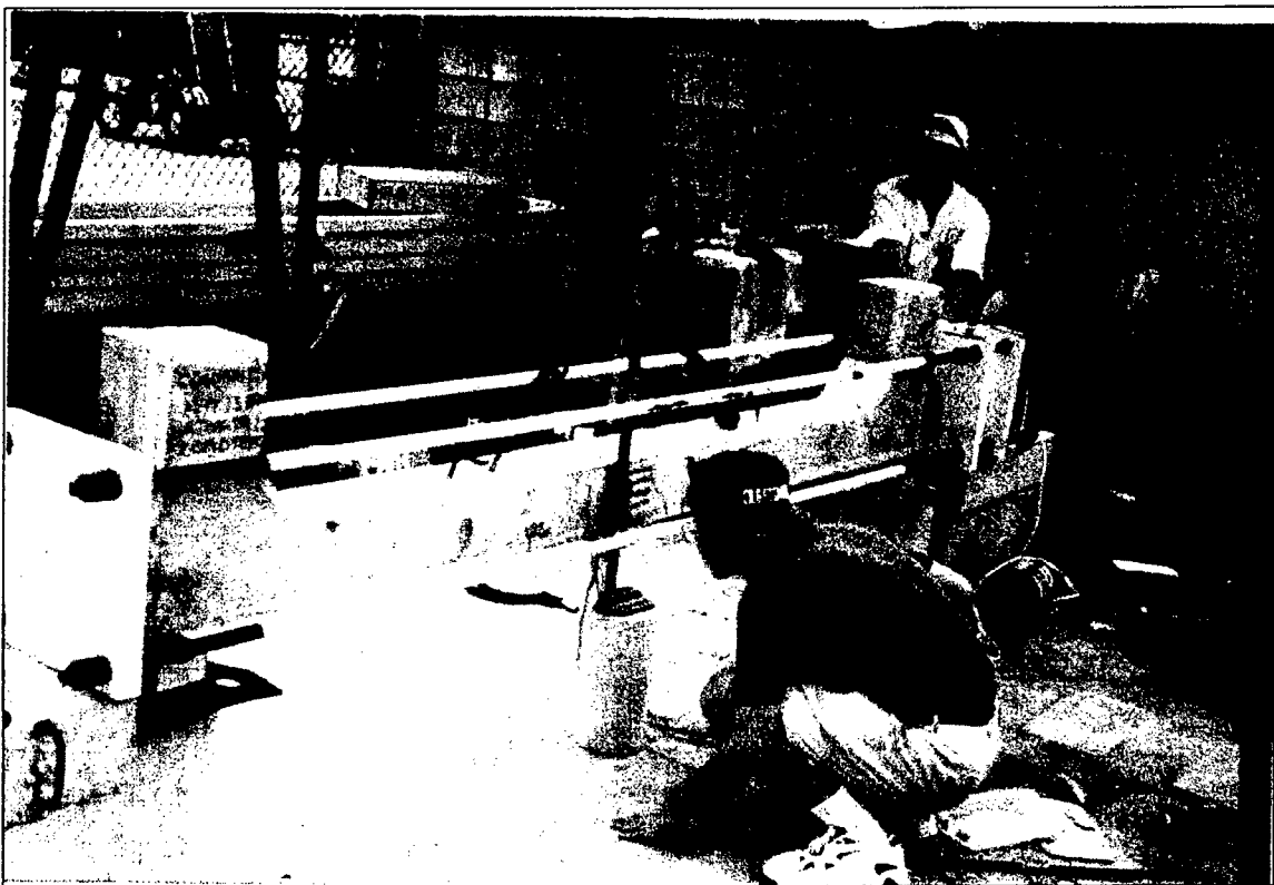
Fig. 5.14 Overview of the steel reaction frame
