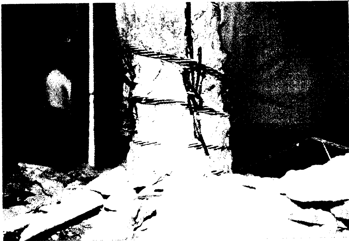
Figure 12.10 View of fractured hoop near the damaged area
