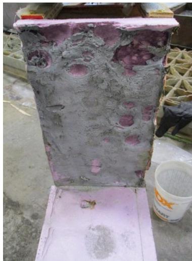
Photo 7.5. Incompatibility of materials.
