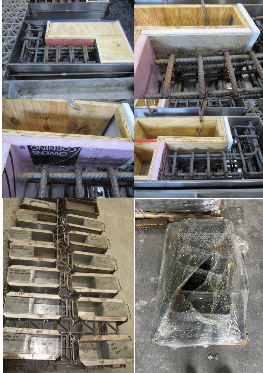
Photo 2.5. Large order of Gr60 rebar, steel formwork, lumber, foam, and associated hardware.
