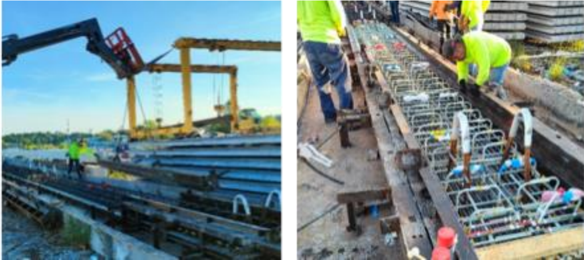
Figure 3-19. Side form installation
