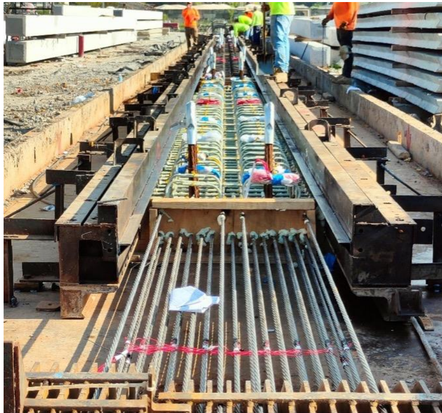
Figure 3-20. FSB forms with reinforcement in place are ready for concrete casting
