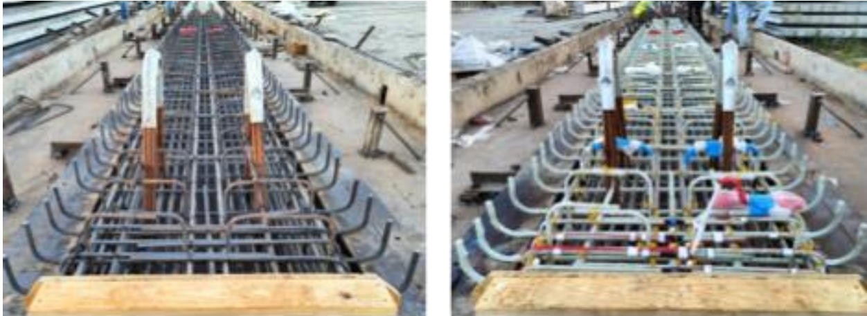
Figure 3-17. Transverse reinforcement, placed and tied
