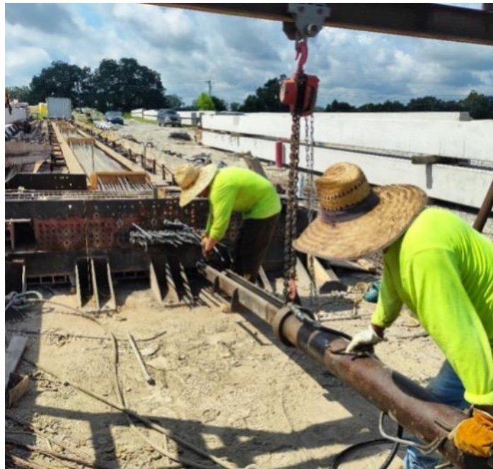
Figure 3-10. Tensioning the strands
