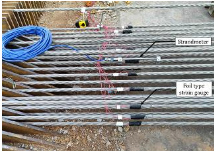
Figure 3-26. Strandmeter and strain gauges installed at the free length
