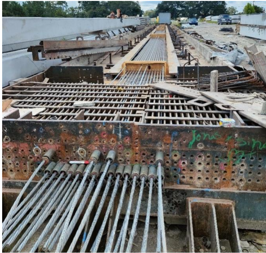
Figure 3-11. Strands are tensioned initially
