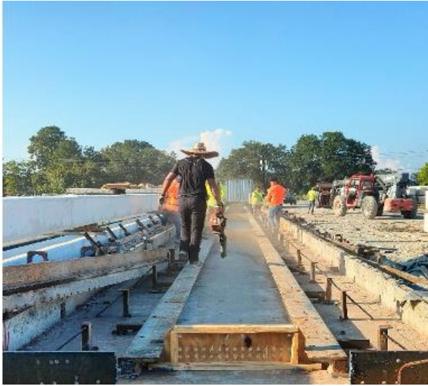
Figure 3-6. Casting bed preparation
