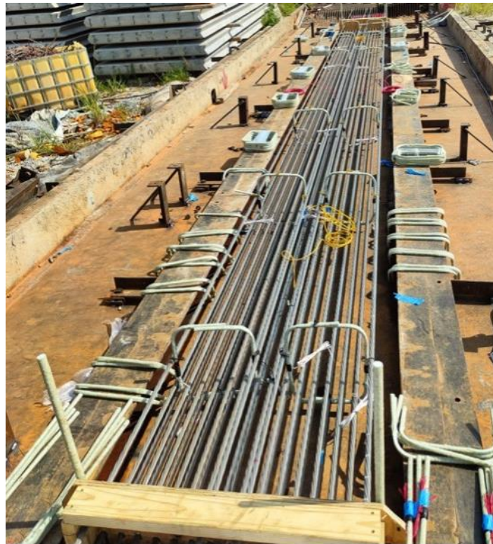
Figure 3-16. Instrumented GFRP K-pairs placed and tied in FSB-4
