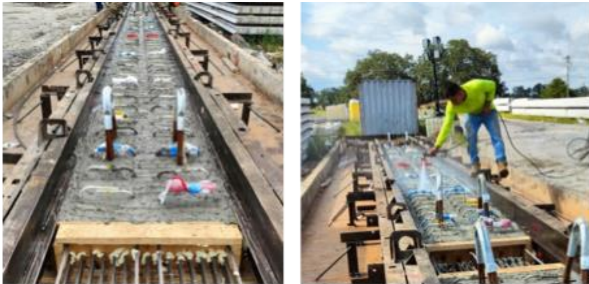
Figure 3-23. Concrete surface finish
