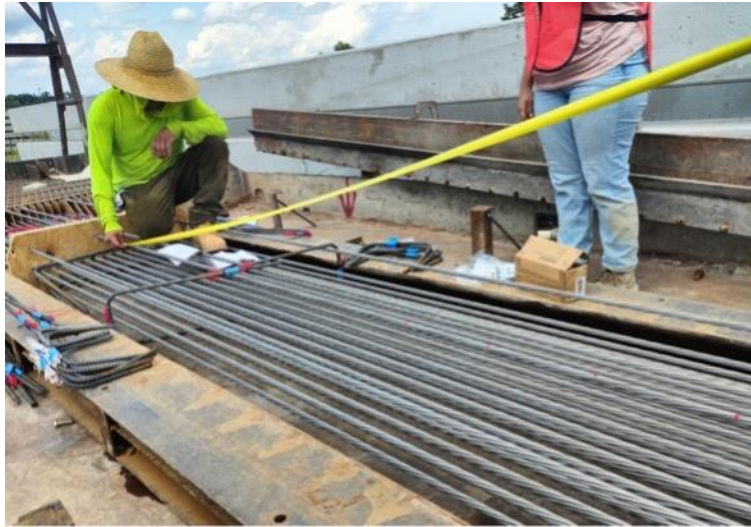
Figure 3-15. Marking and placing the instrumented D-pairs at FSB-1
