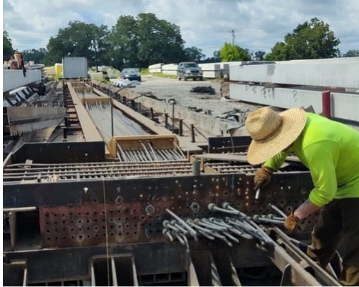
Figure 3-8. Seated strands in the chucks
