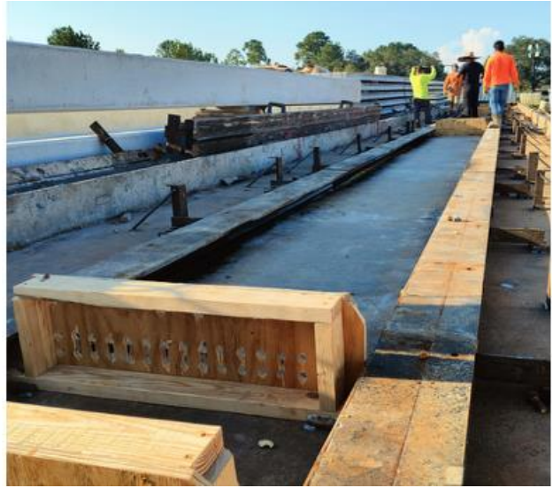
Figure 3-6. Casting bed preparation
