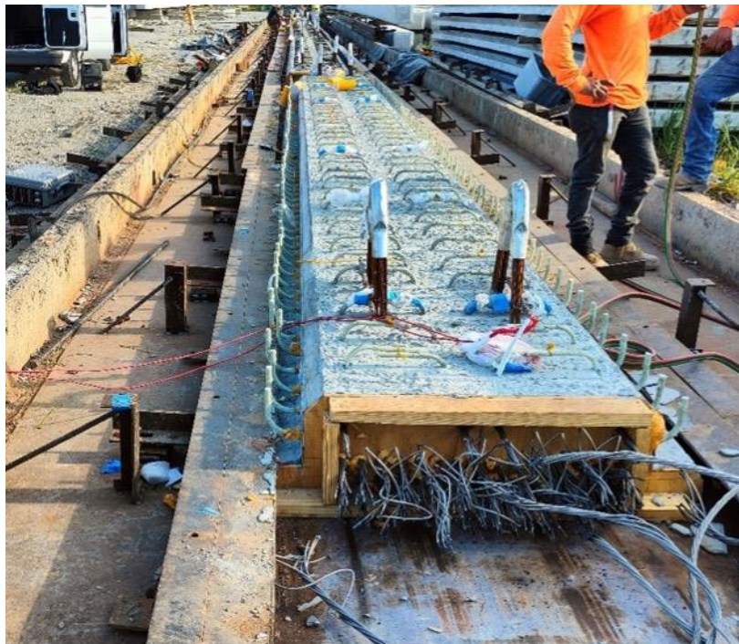
Figure 3-31. End 8 after rupture
