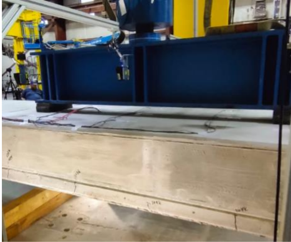
Figure 10-17. Flexural cracks at bottom flanges
