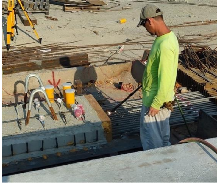
Figure 3-28. Strand cutting at End 1
