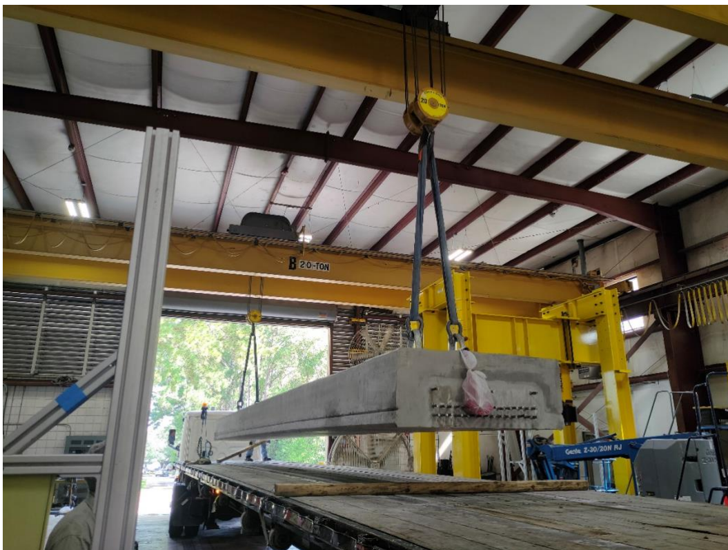
Figure A5-2. Lifting FSB 4 from the truck
