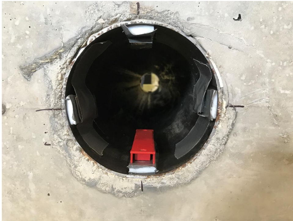
Figure 4.18 Teflon strips positioned within the steel guide tubes with magnets to hold them in place while the adhesive sets
