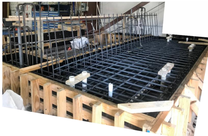
Figure 5.6 Reinforcing bars positioned inside deck formwork
