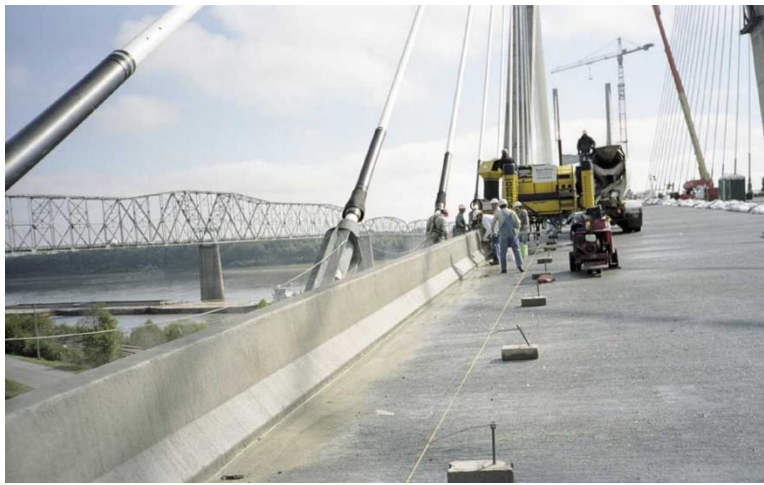
Figure 1.1 Slip-formed concrete traffic railing (Photo credit: Gomaco)
