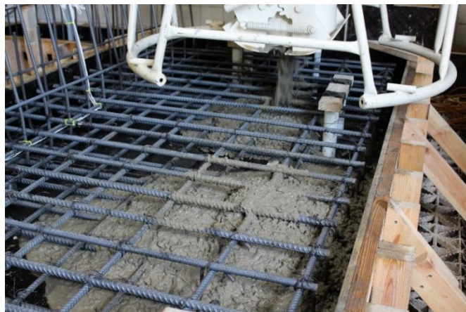
Figure 5.8 Deck concrete placement
