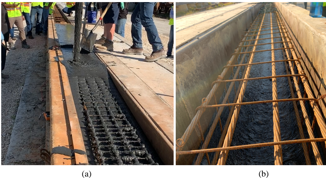
Figure 3: 18-in. square UHPC pile fabrication showing (a) concrete pouring at one end, and (b) concrete self-consolidating at the other end.
