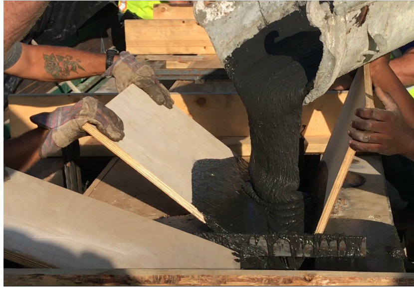
Figure 4: Concrete pouring into the H-Pile forms
