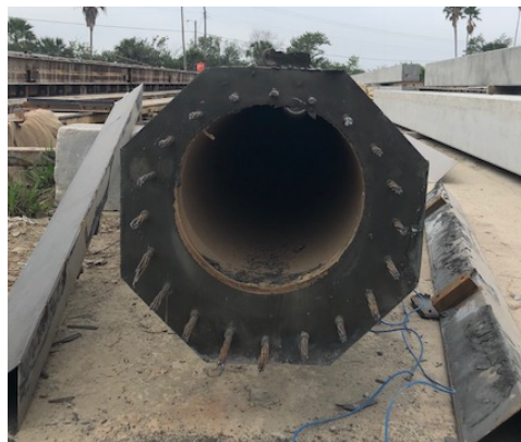
Figure 7: Voided 24-inch octagonal UHPC pile after removal of forms
