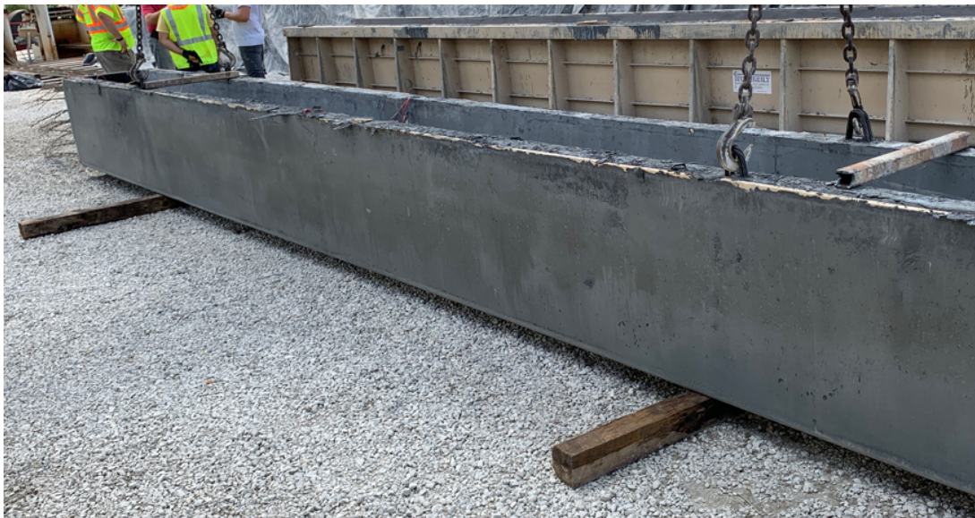
Figure 5: H-Pile after removal of forms
