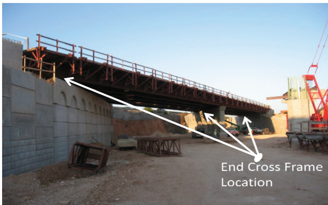
Figure 1.18 60° Skewed Steel Bridge in Lubbock, TX with End Cross-frames[31]
