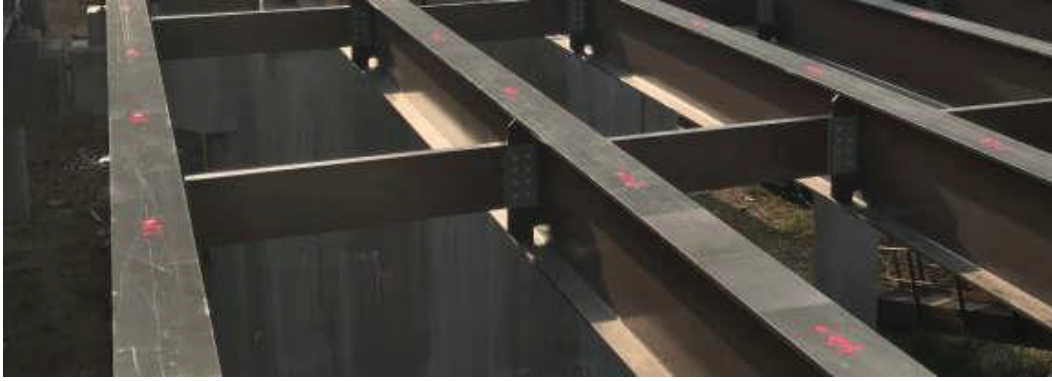
Figure 1.11 Diaphragm in Steel Girder Bridges
