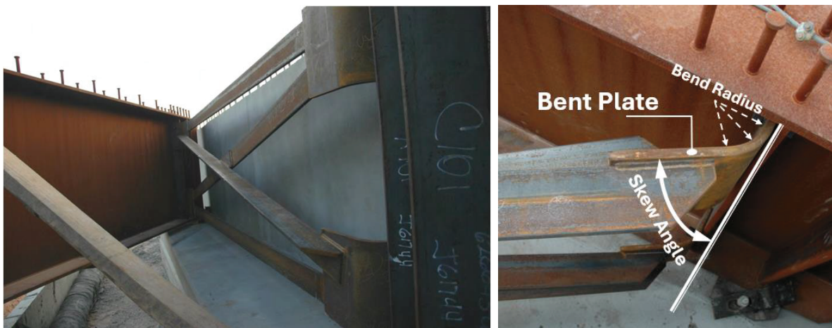
Figure 1.36 Bent plate end cross-frame connection[45]
