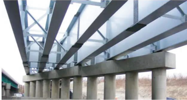
Figure 1.3 A skew bridge under construction (Roads & Bridges, November 2015)
