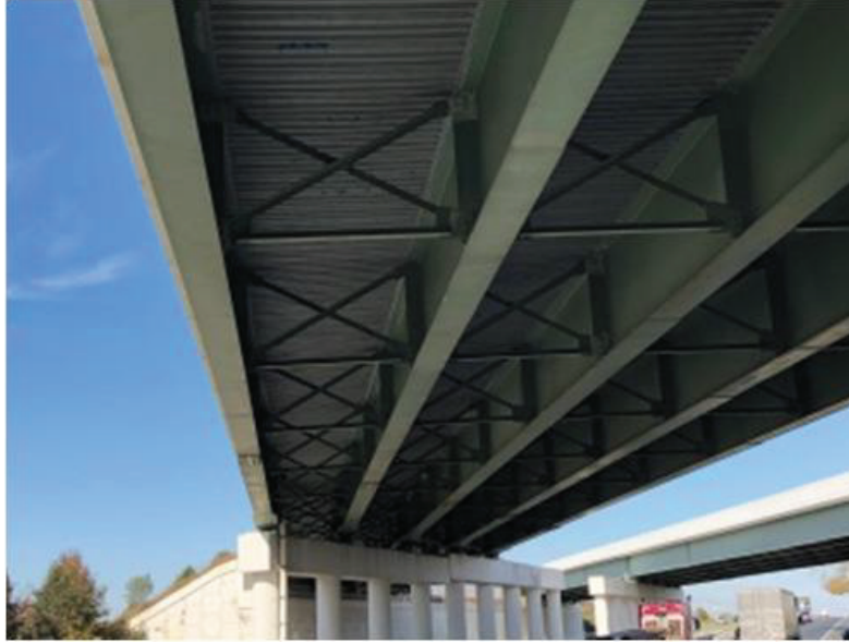
Figure 1.7 X- shape Cross-frame in Steel Girder Bridges[23]
