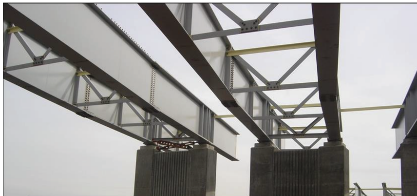
Figure 1.9 K-type Cross-frame in Steel Girder Bridge
